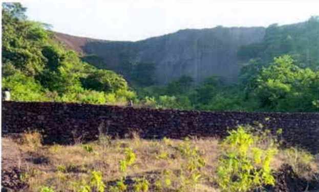
LBRW to retain runoff and replenish groundwater
