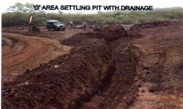
Trenches dug near G-Area for Rainwater Harvesting
