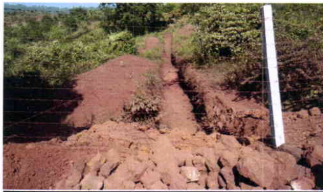
Contour bunds created to trap rainwater for harvesting.
