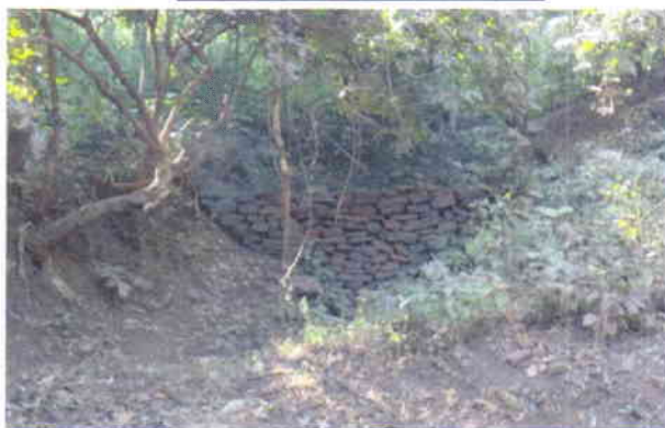
Gully plugs installed at various junctures to arrest rainwater
