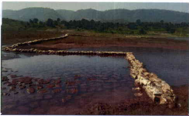
Sandbag Checkdam near Tailing Pond to prevent flow Turbid water.
