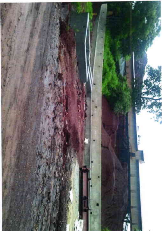
Settling Pit with Garland Drain surrounding DH-5 Dump.
