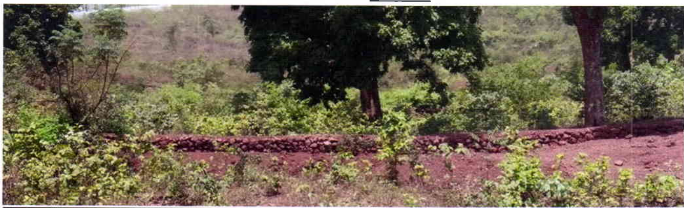
LCBDs at Eco-Restoration site catering partially to watering requirements for the plantation in site
