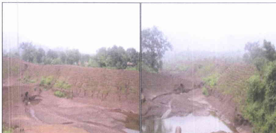
Photograph: Vetiver Plantation to bind the Soil at Slope of Sedimentation Traps
