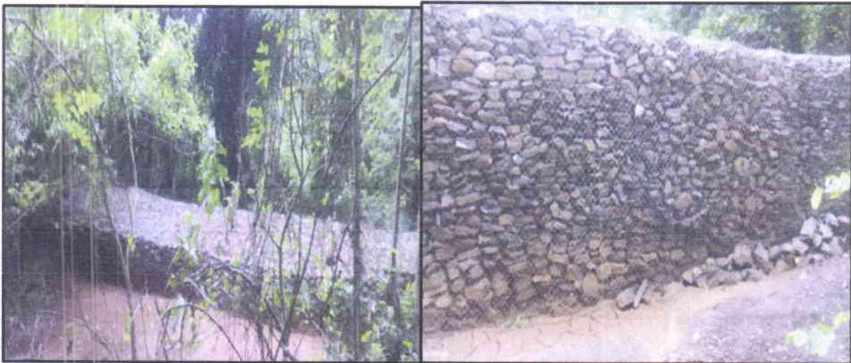
Photograph 3: Newly Constructed Boulder Wall at OT Hill Waste Dump Area
