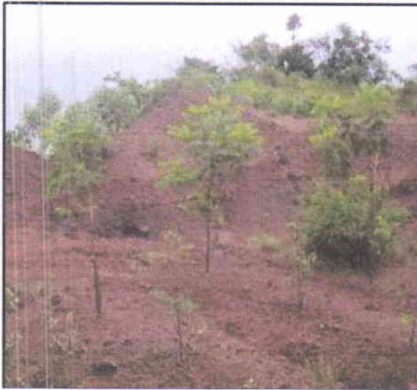
Photograph 1: Stabilized Old Waste Dump
