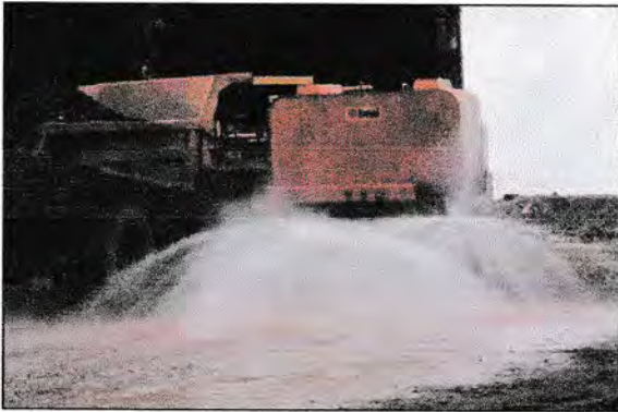
Photograph 1: Haul Road Water Sprinklers
