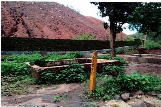
GARLAND DRAIN AROUND WASTE DUMP
