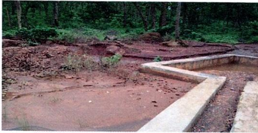
SILT CATCHMENT DRAIN NEAR WASTE DUMP WATER RECHARGE PIT
