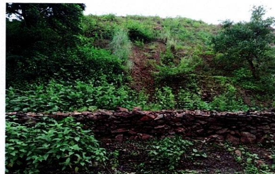
COIR MAT WITH VERTIVER GRASS STABILIZING DUMP
