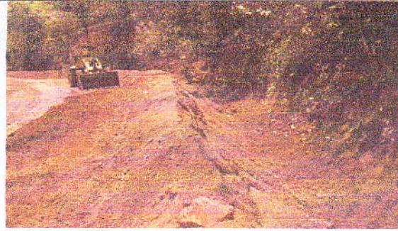
Drainages are cleaned to stop overflow of silt
