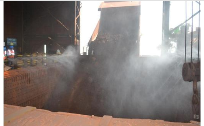
Photograph showing High Pressure Dust suppression installed at Feed Hopper at Hill Top Plant
