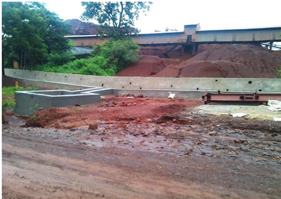
Settling Pit with Garland Drain surrounding DH-5 Dump.
