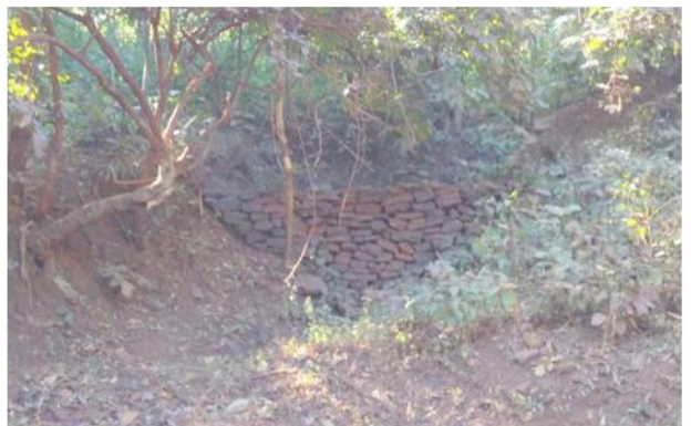
Gully plugs installed at various junctures to arrest rainwater
