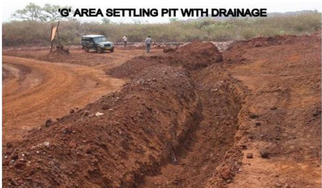
Trenches dug near G-Area for Rainwater Harvesting
