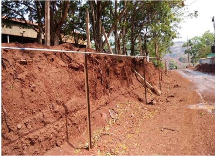
Photograph showing Fixed water sprinkling system on Haul Road from Panposh
