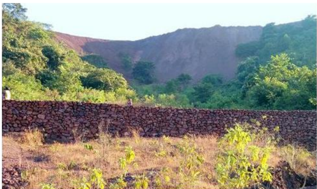
LOBRW to retain runoff and replenish groundwater
