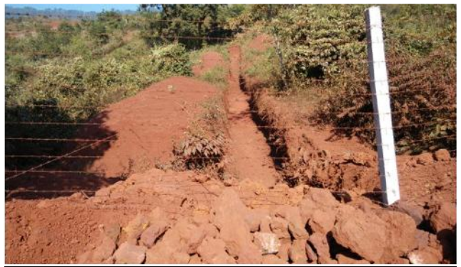
Contour bunds created to trap rainwater for harvesting.
