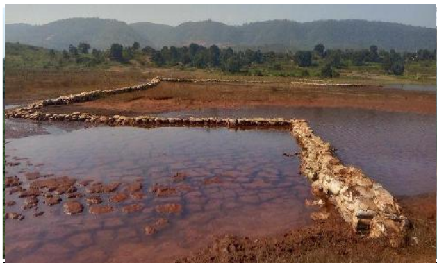
Sandbag Checkdam near Tailing Pond to prevent flow of Turbid water.
