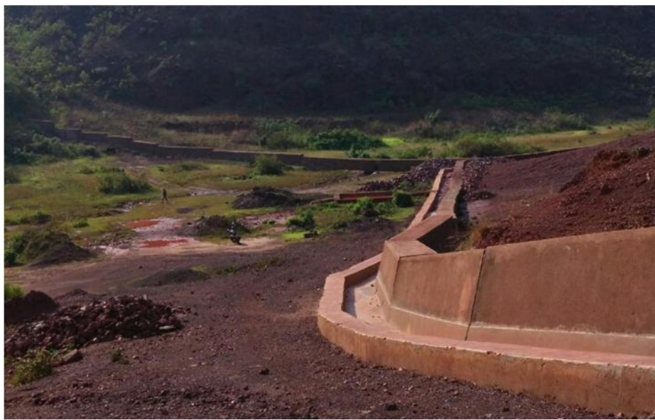
Retaining Wall with Garland Drain around Panposh OB Dump
