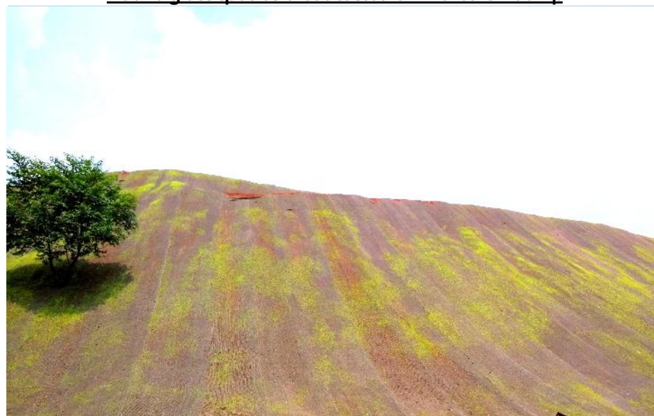
Coir Matting on DH-5 subgrade dump
