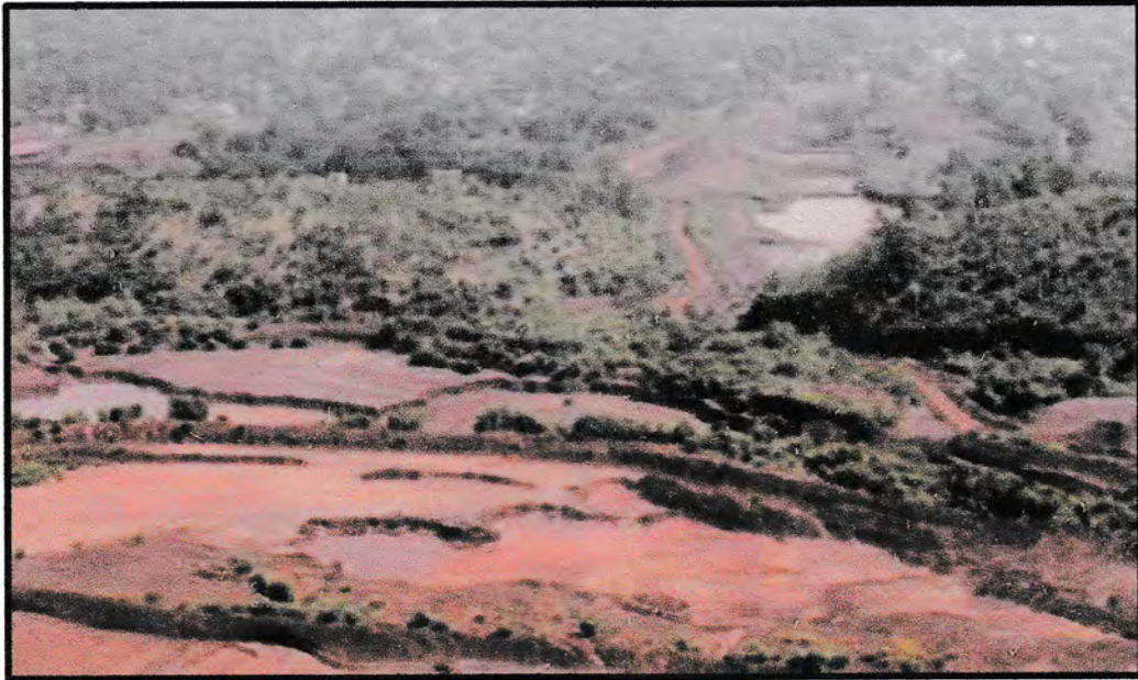
Photograph 1: Dams at the slope of Fines Heap (Dams 1- 5)& 04 no.s' of Sedimentation Traps
