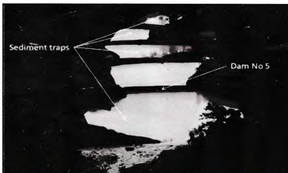
Photograph 2: Check Dams and Settling Pits / Sediment Traps constructed to control flow of fines
