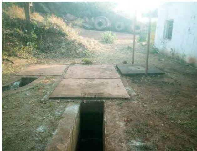
Oil & Grease trap at F/M Area, Barsua
