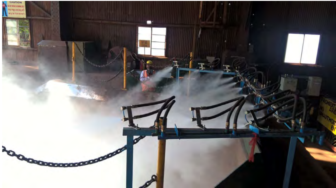
Dry fog system at Crusher, Barsua
