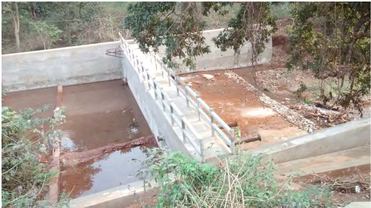
Check dam constructed across the overflow channel of tailing dam to re-cycle the water, Barsua
