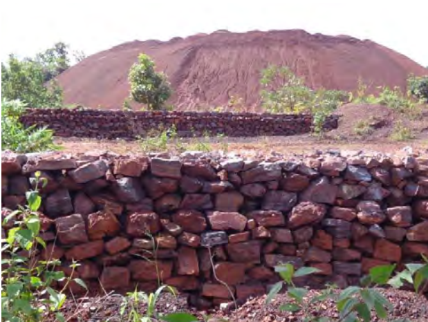
Retaining wall at Sub-grade dump at Barsua
