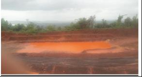
A sump prepared in M3 area for collection of rain water and ground water recharging
