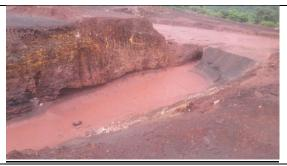
A Sump prepared in M3 area to arrest the flow of silt and sediment
