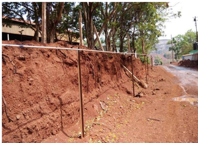
Photograph showing Fixed water sprinkling system on Haul Road from Panposh
