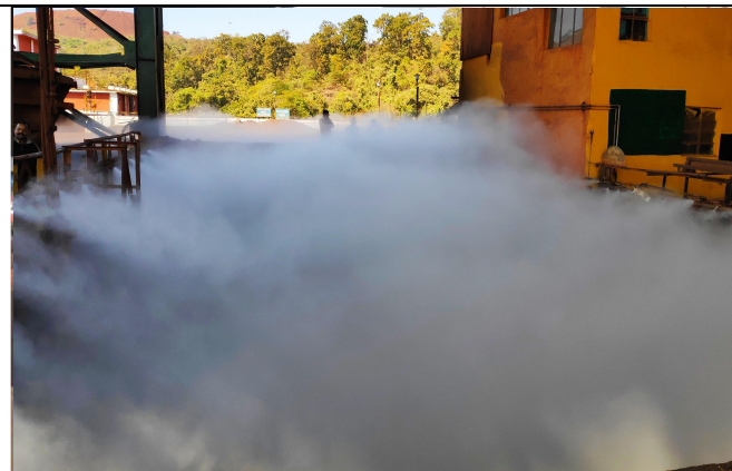
Photograph showing Dry Fog Dust suppression System installed at Feed Hopper at Hill Top Plant
