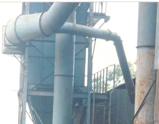
Photograph showing Bag House installed at secondnary Crushing Point
