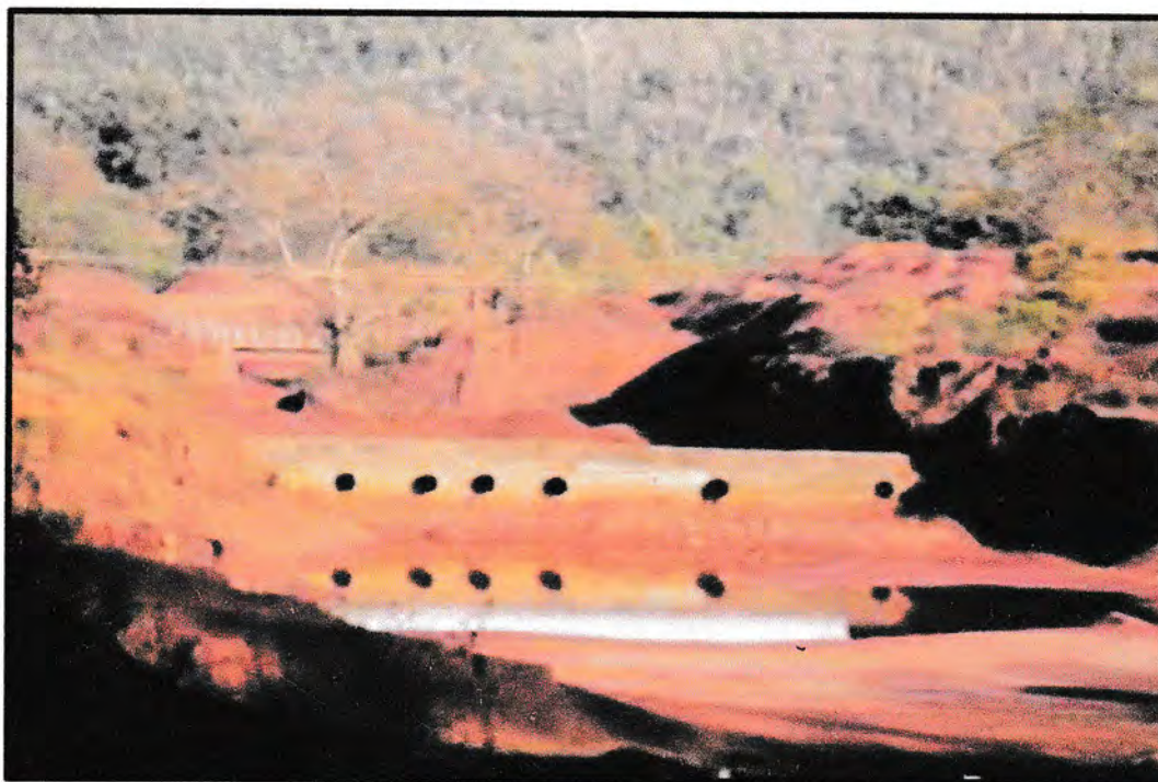
Photograph 2: Concrete Check dam at Dam No.5 following four nos. of Sedimentation Traps towards zero point nalla
