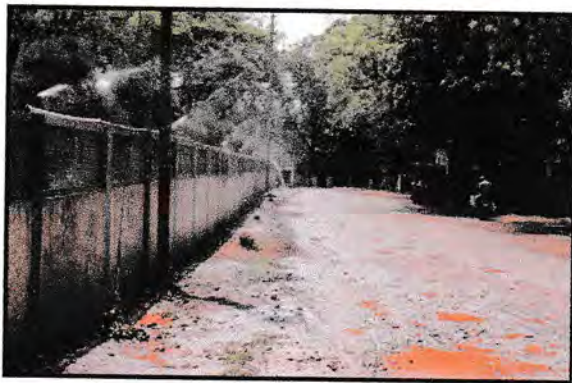
Photograph 3: Permanent Road Sprinklers in Township
