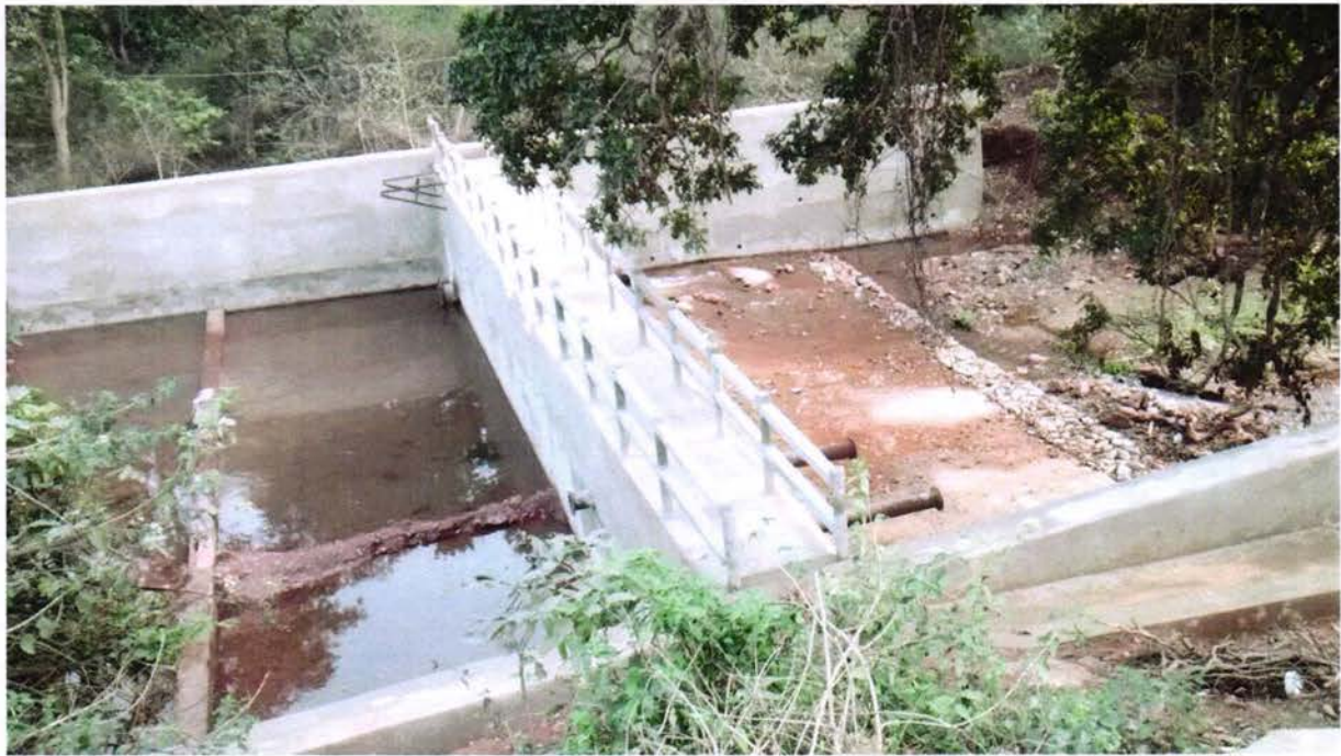
Check dam constructed across the overflow channel of tailing dam to re-cycle the water, Barsua
