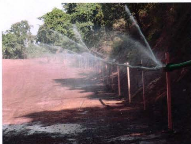
Fixed sprinkler at Crusher, Barsua
