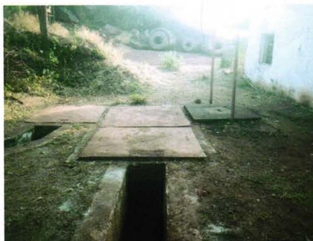
Oil & Grease trap at F/M Area, Barsua
