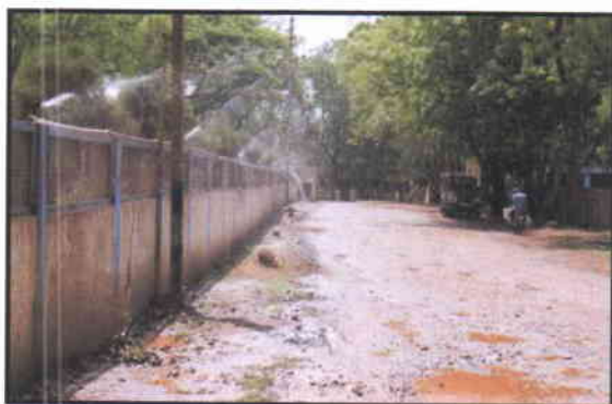
Photograph 3: Permanent Road Sprinklers in Township
