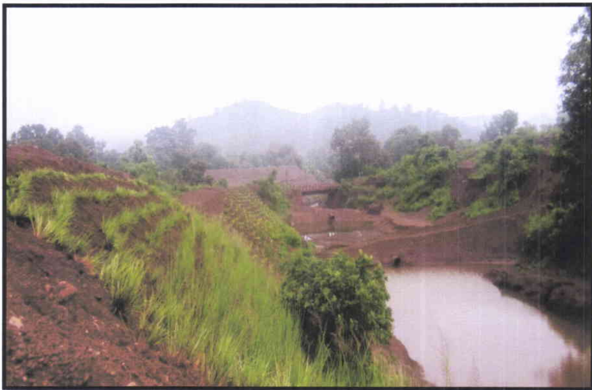
Photo: Settling cum Harvesting Pits along-with vetiver plantation near Zero Point Nalla
