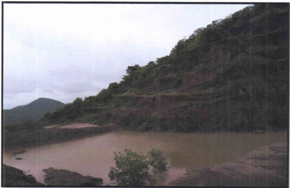
Photo: Rain Water Harvesting Cum Settling Pond at Bai Hill Area of Mines
