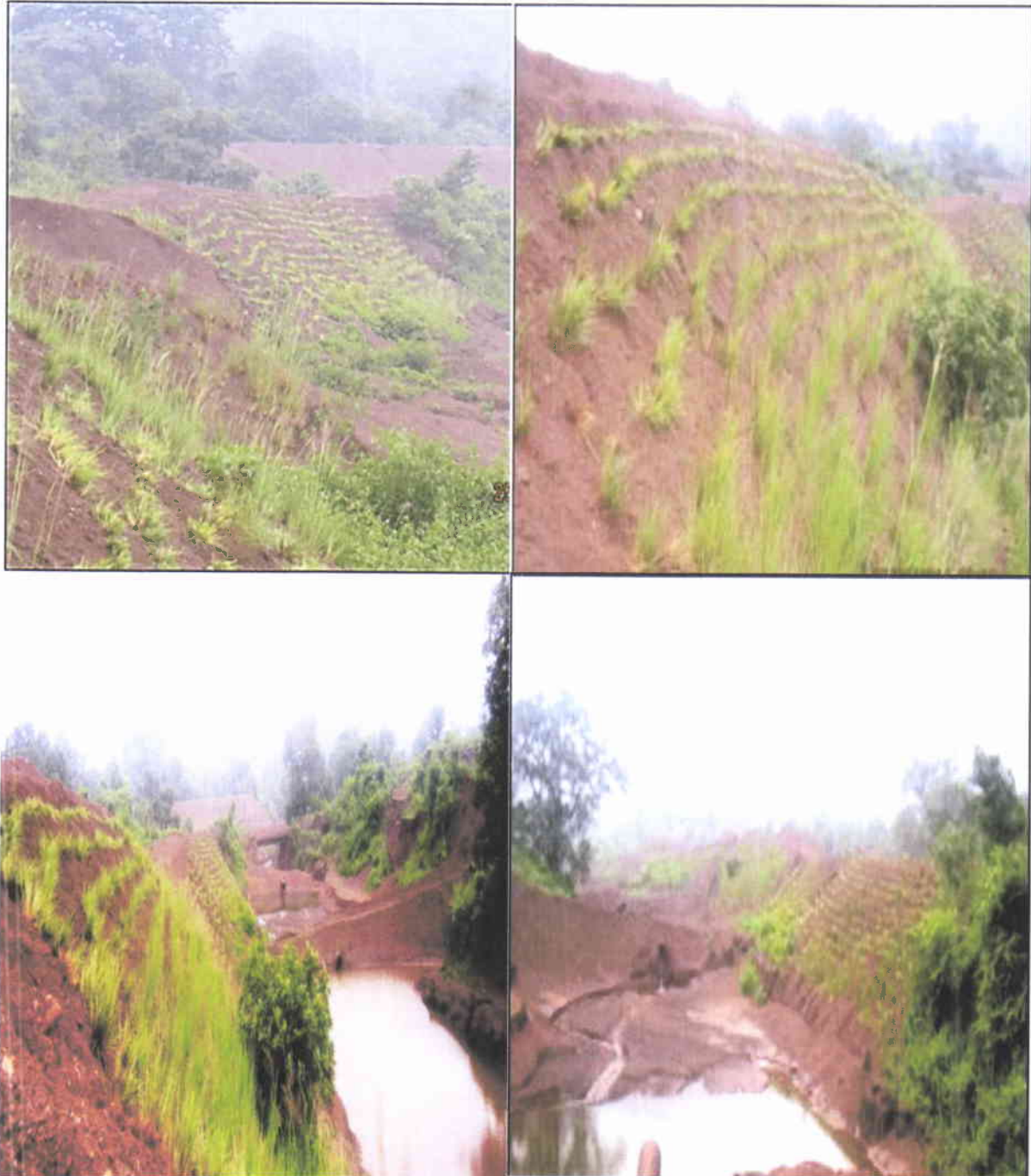
Photograph: Vetiver Plantation to bind the Soil at Slope of Sedimentation Traps
