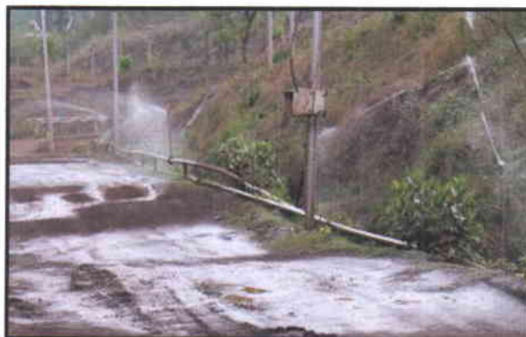
Photograph 2: Permanent Road Sprinklers in Mines
