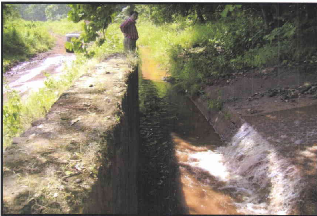
Photo: Garland Drain to divert runoff water into the pits
