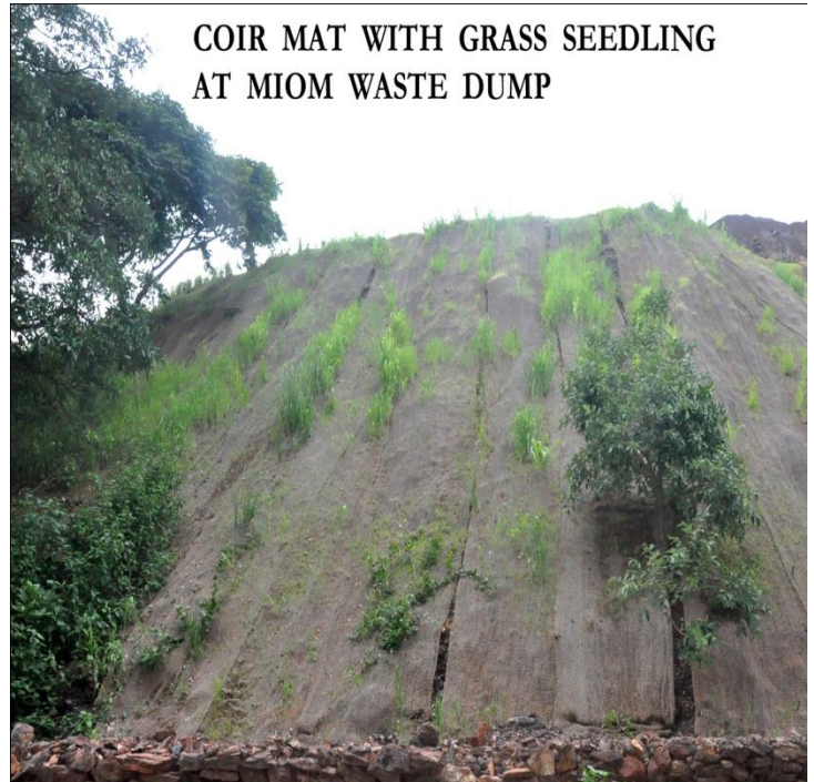
Coir Mat over waste dump slope
