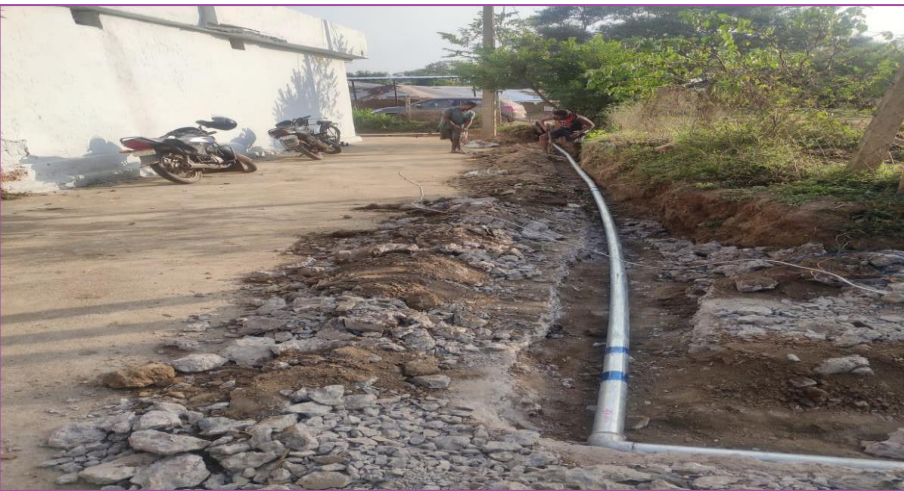
Pipeline work for drinking water ( Mahakakala )
