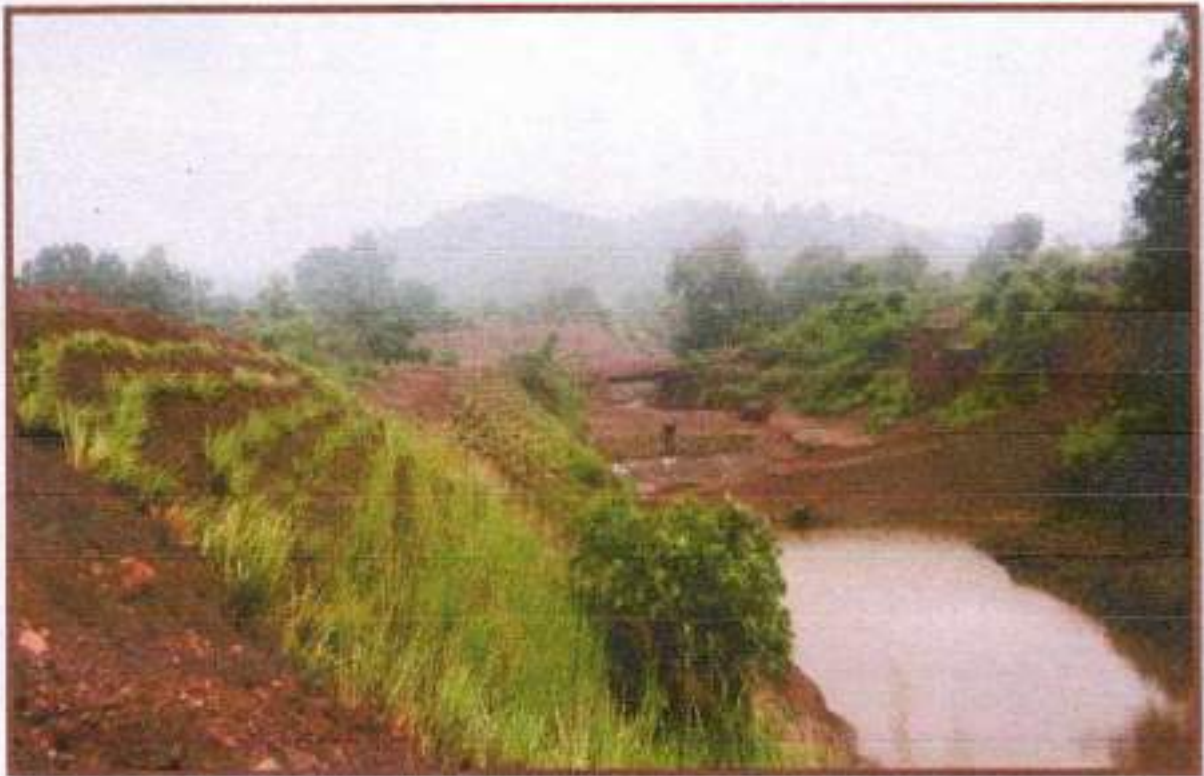
Photo: Settling cum Harvesting Pits along-with vetiver plantation near Zero Point Nalla
