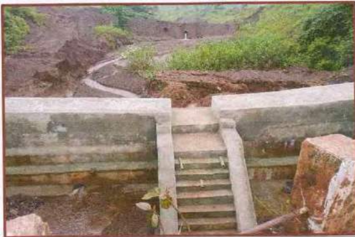
Photo: Concrete check dam at Zero point area
