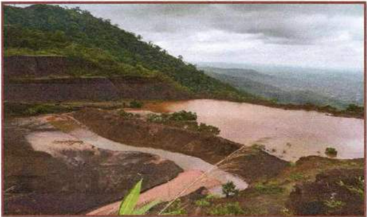
Photo: Rain Water Harvesting cum Settling Pond at IInd Level Area of Mines
