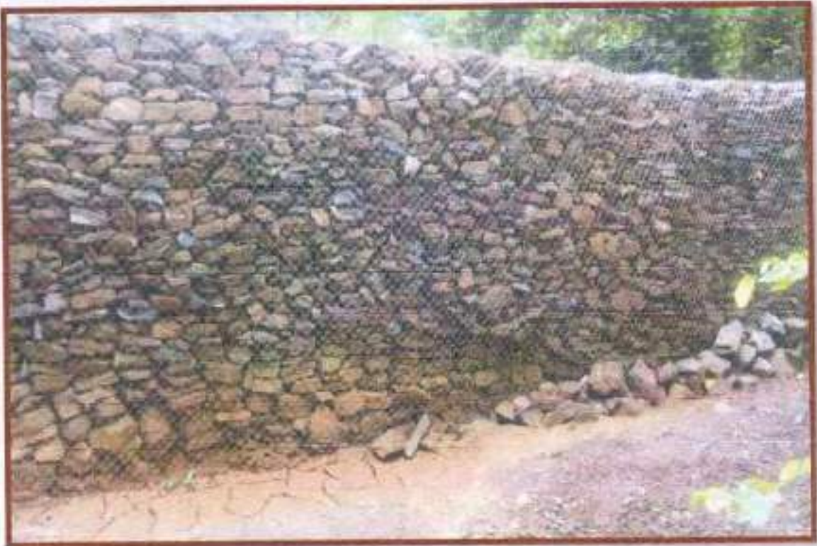
Photo: Boulder Wall the bottom of OT Hill Waste Dump
