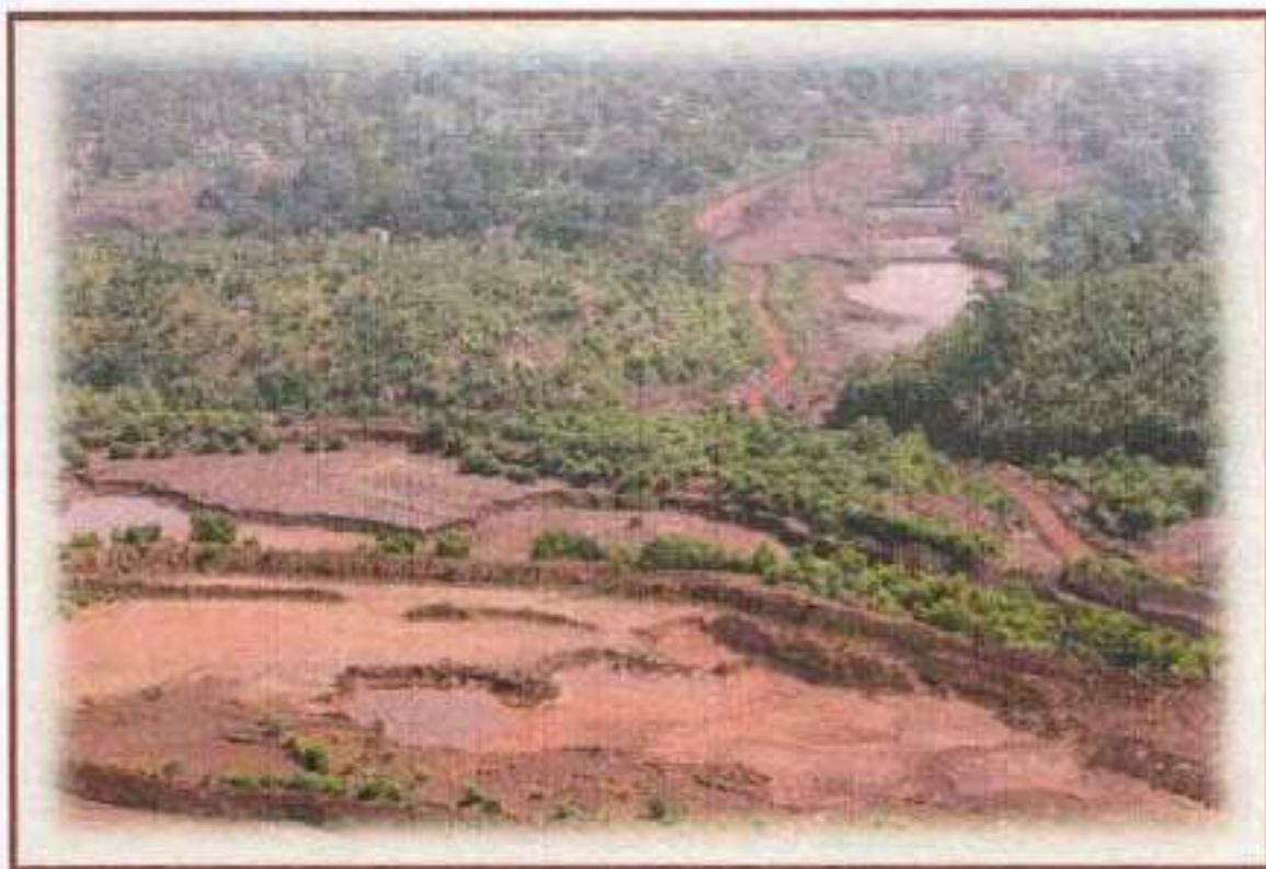
Photo: Earthen Dams and Sedimentation Traps at the slope of Fines Heap
