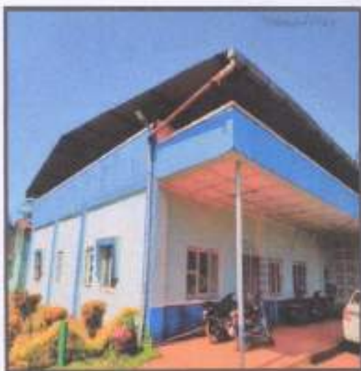
ANNEXURE-17: A- ROOFTOP RAINWATER HARVESTING SCHEME INSTALLED AT KIOM GENERAL OFFICE SHOWING COLLECTION, KIOM, SAIL
