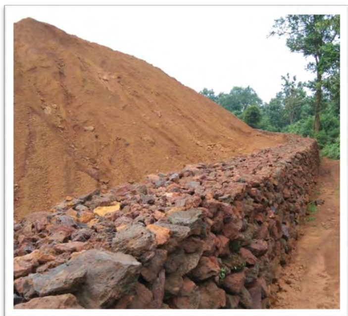
Retaining wall at Waste dump No. -2
