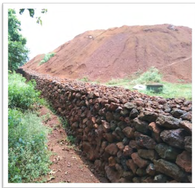
Retaining wall at Waste dump No. -2
