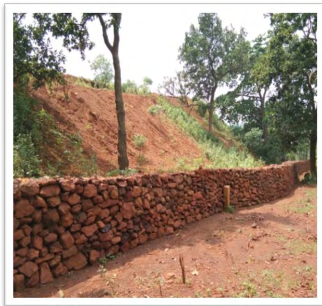
Retaining wall at Waste dump No. - 1
