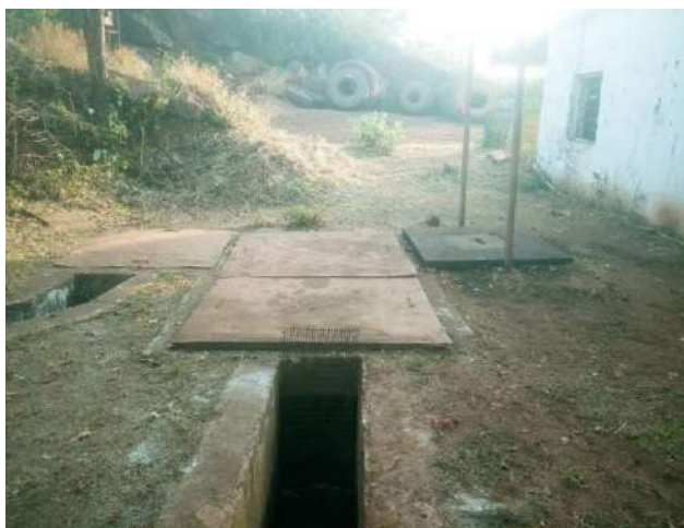
Oil & Grease trap at F/M Area, Barsua
