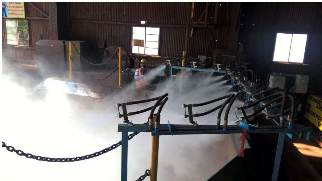
Dry fog system at Crusher, Barsua
