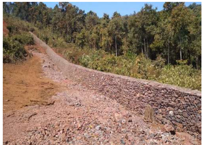
Dry Boulder wall at Waste Dump, Taldih
