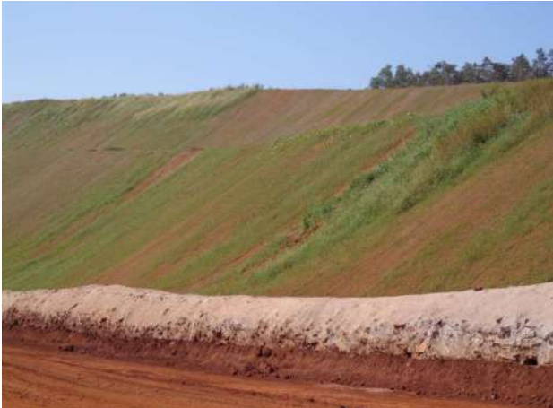
Coir mating over the dump at Barsua
