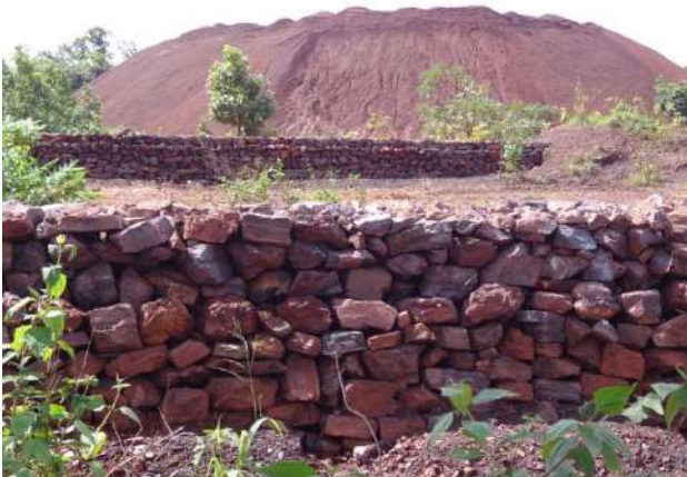
Retaining wall at Sub-grade dump at Barsua
