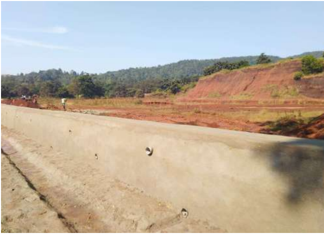
Retaining wall around tailing stockyard
