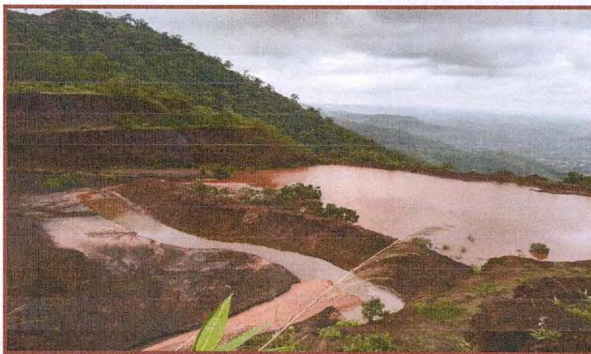
Photo: Rain Water Harvesting cum Settling Pond at IInd Level Area of Mines
