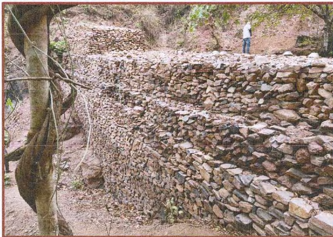
Photo: Boulder wall constructed at the toe of Ranichua waste dump area
