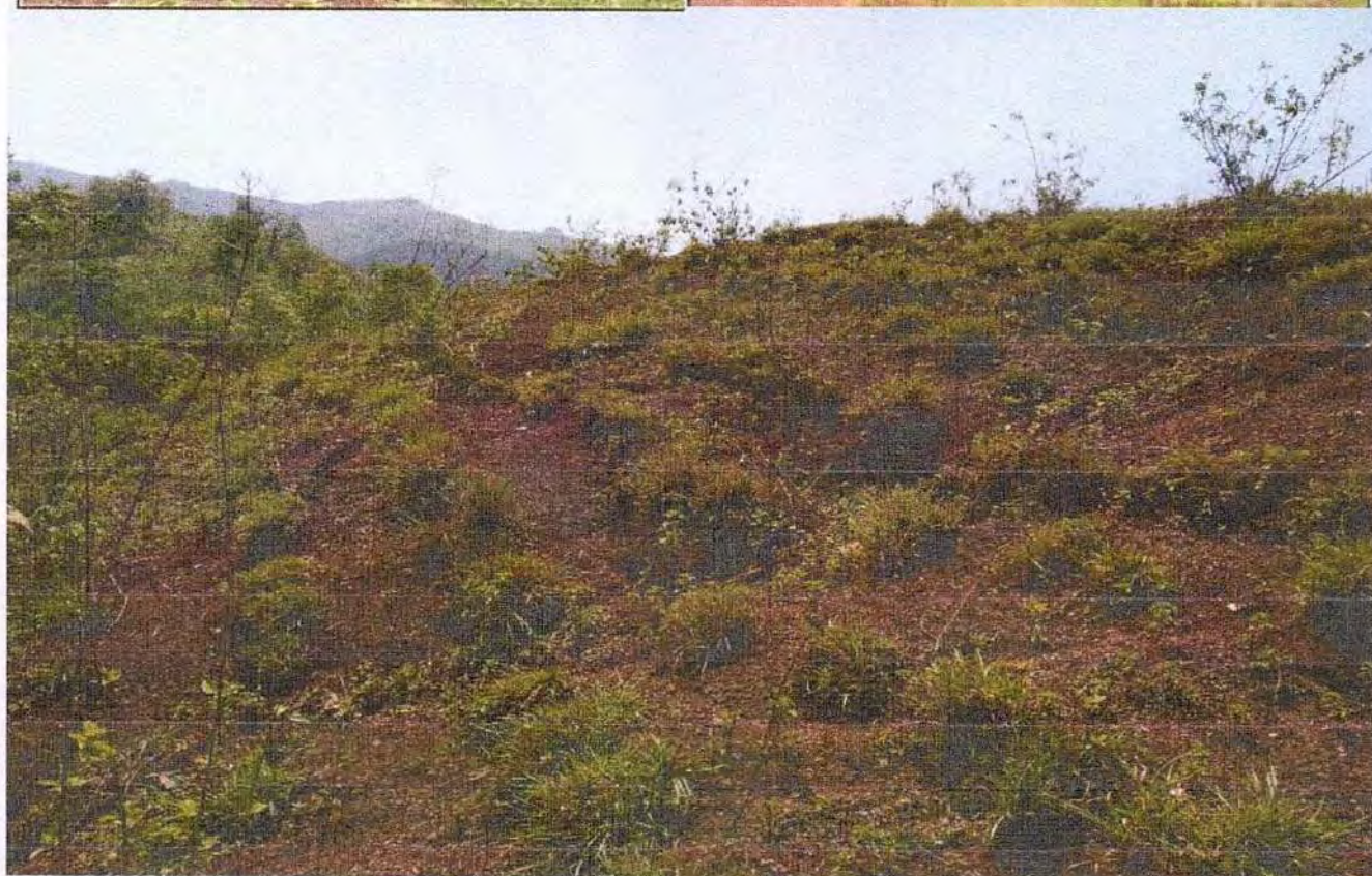
Photograph: Vetiver Plantation to bind the Soil at Slope of Sedimentation Traps
