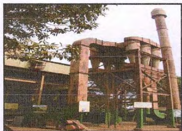
Photograph 6: Dust Extraction System at Crushing Plant
