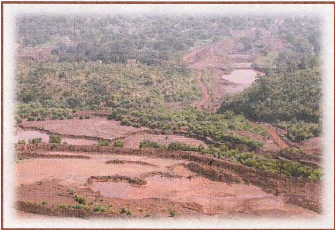
Photo: Earthen Dams and Sedimentation Traps at the slope of Fines Heap
