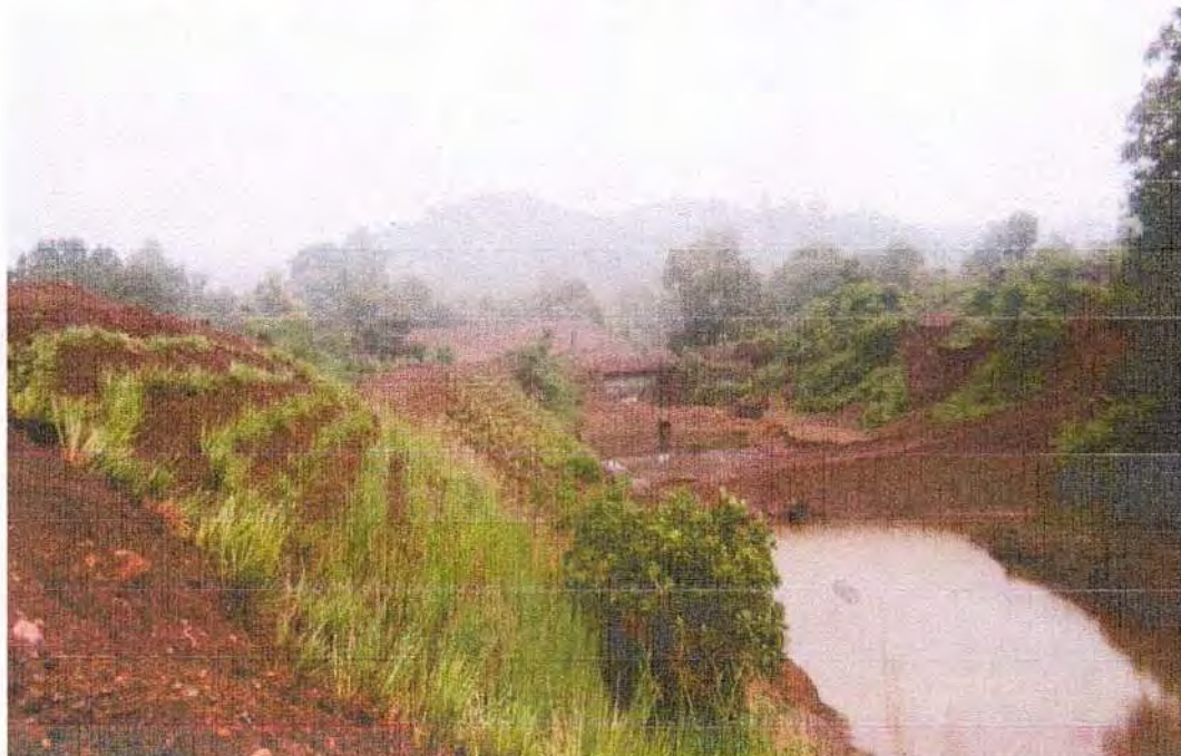
Photograph 2: Check Dams and Settling Pits / Sediment Traps constructed to control flow of fines
