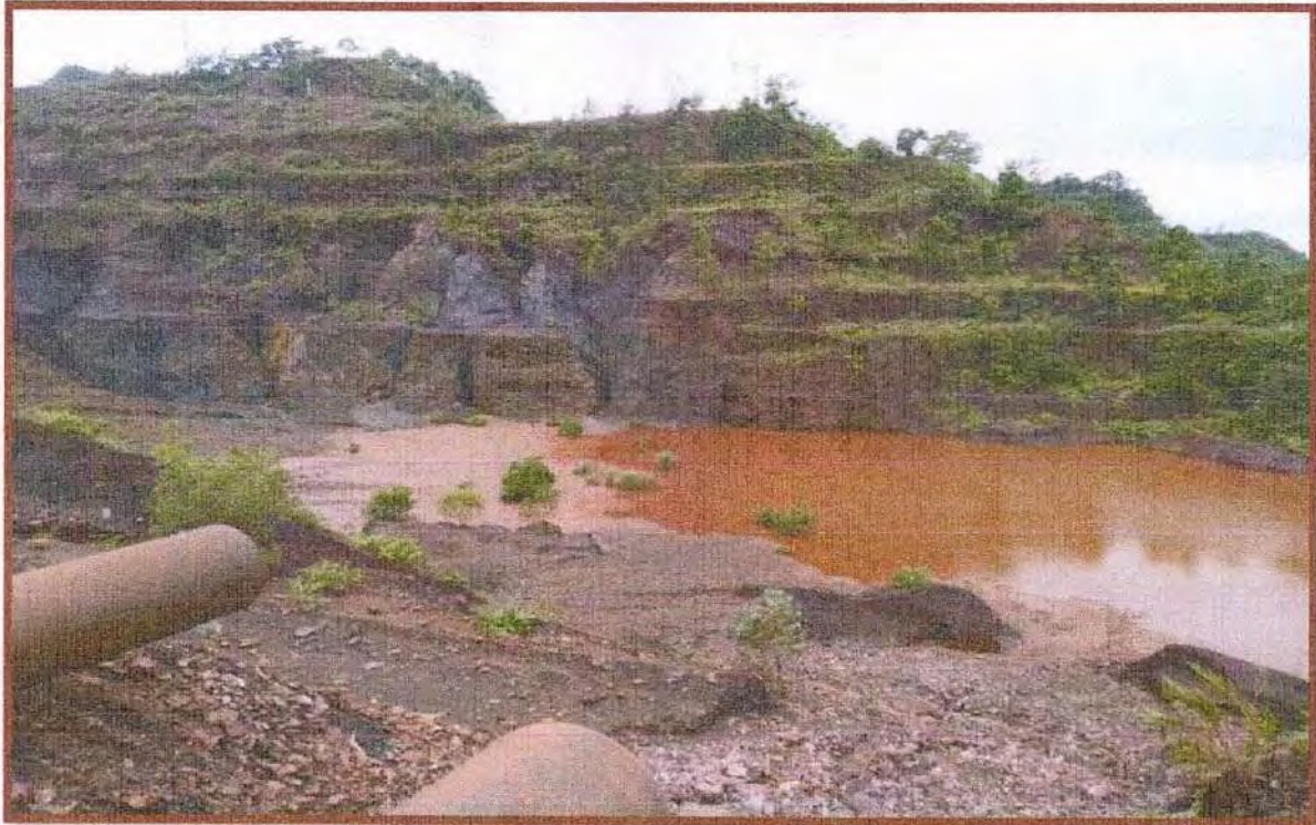
Photo: Rain Water Harvesting Cum Settling Pond at HD Buru Area of Mines
