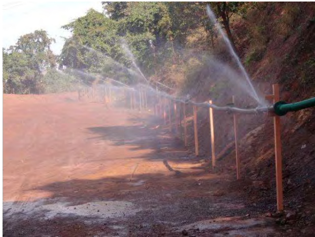
Fixed sprinkler at Crusher, Barsua
