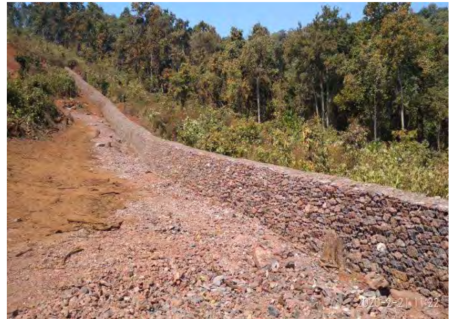
Dry Boulder wall at Waste Dump, Taldih
