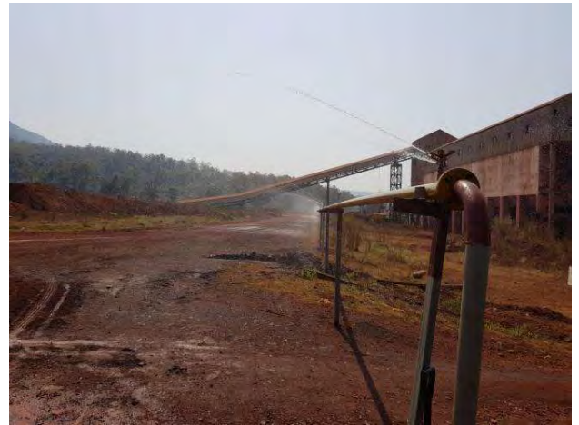
Fixed Sprinkler at Loading Plant, Barsua
