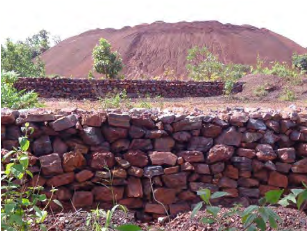
Retaining wall at Sub-grade dump at Barsua
