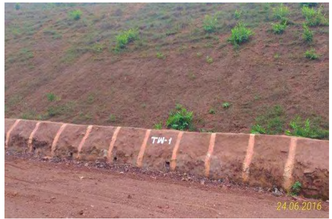
Tow wall at the bottom of Dump-8, Barsua
