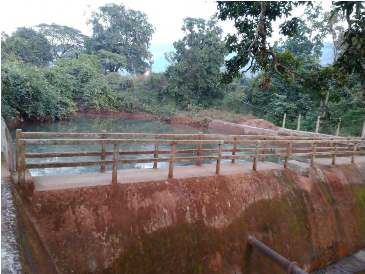
Check dam constructed across the overflow channel of tailing dam to re-cycle the water, Barsua
