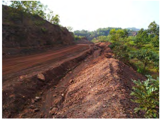
Garland drains to channelized the water towards Area 3E pit
