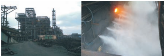
Coke Dry Cooling Plant at ISP
