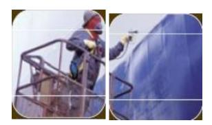
Sheeting work are to be done with cordless gun for fixing the self tapping screwed depending upon availability & site requirements. MEWP /man lifters are to be used for access.
