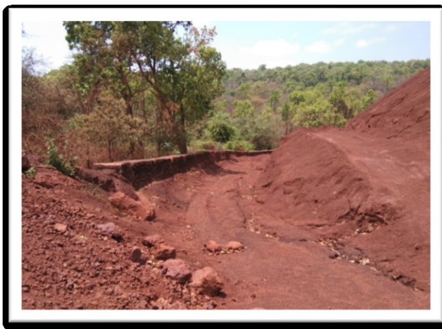
Garland Drain at Sub grade Dump
