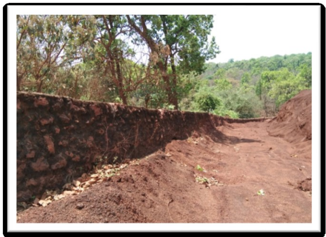
Garland Drain at Sub grade Dump
