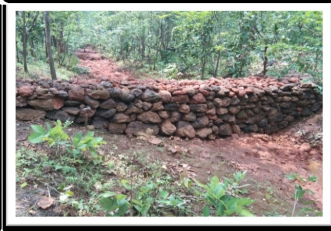
Check Dam constructed during July -20 & Aug -20
