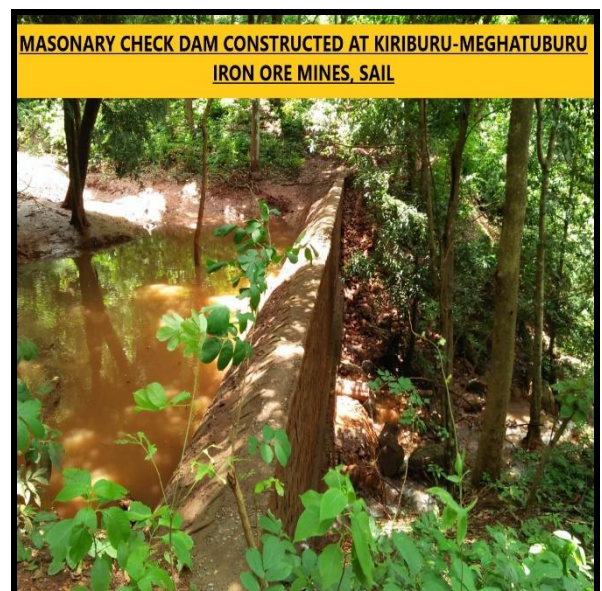
ANNEXURE-19: D- MASONARY CHECK DAM CONSTRUCTED AT KIRIBURU-MEGHATUBURU IRON ORE MINES, SAIL
