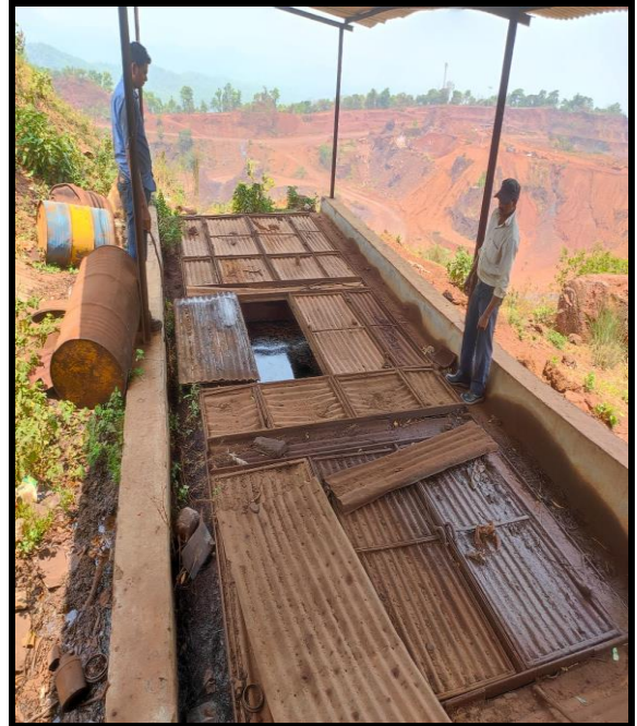
ANNEXURE-11: B- EFFLUENT TREATMENT UNIT (ETP) - EFFLUENT OIL & GREASE TRAP INSTALLED AT KIOM, SAIL
