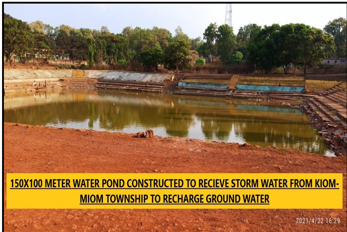
ANNEXURE-16: E- 150X100 METER WATER POND CONSTRUCTED TO RECIEVE STORM WATER FROM KIOM-MIOM TOWNSHIP TO RECHARGE GROUND WATER
