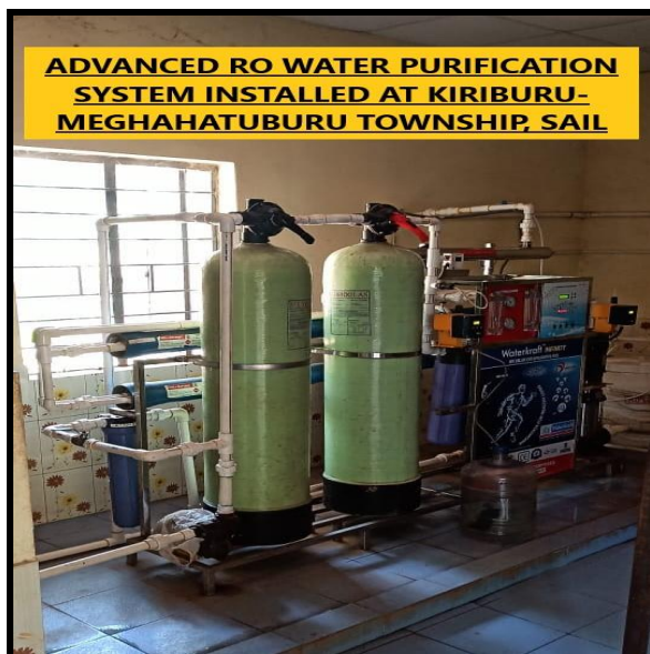
ANNEXURE-3: B- ADVANCED RO WATER PURIFICATION SYSTEM INSTALLED AT KIRIBURU-MEGHAHATUBURU TOWNSHIP UNDER THE CSR SCHEME OF MEGHAHATUBURU IRON ORE MINES, SAIL
