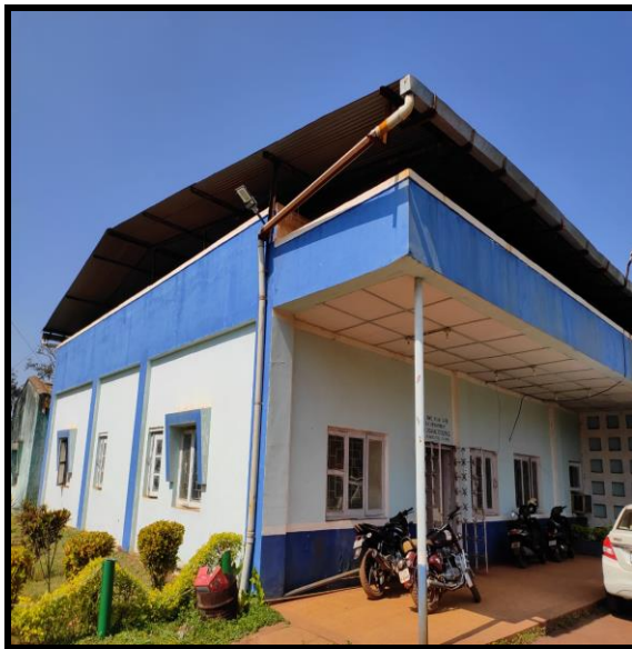
ANNEXURE-16: A- ROOFTOP RAINWATER HARVESTING SCHEME INSTALLED AT KIOM GENERAL OFFICE SHOWING COLLECTION, KIOM, SAIL
