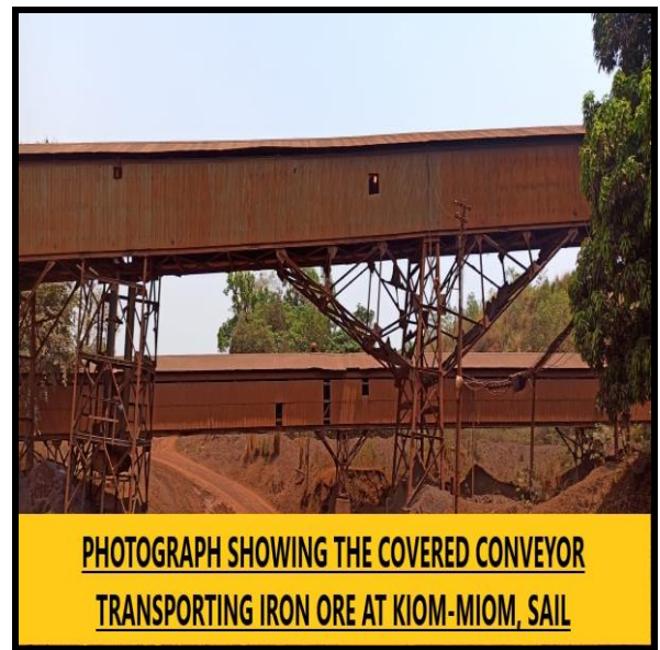
ANNEXURE-7: B- PHOTOGRAPHS SHOWING THE COVERED CONVEYOR TRANSPORTING IRON ORE AT KIOM-MIOM, SAIL
