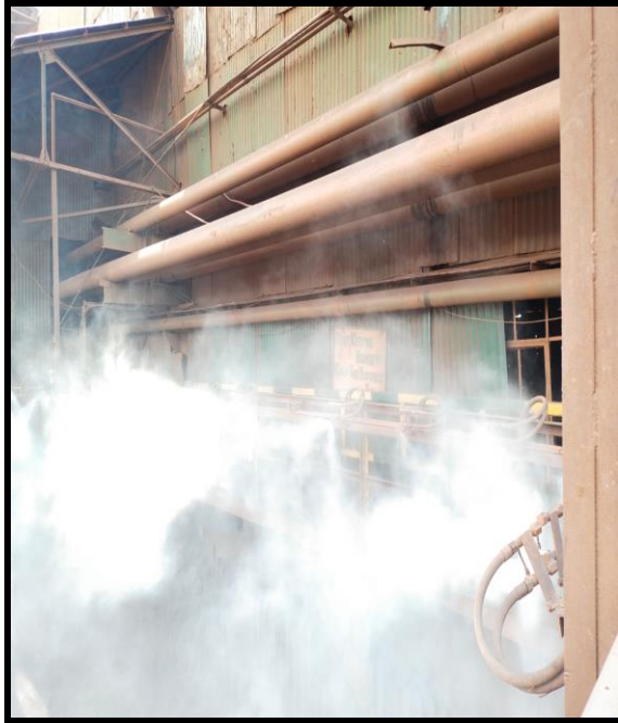
ANNEXURE-8: C- DRY FOG DUST SUPPRESSION SYSTEM INSTALLED AT HOPPER, MINERAL SEPARATION PLANT AT KIOM, SAIL
