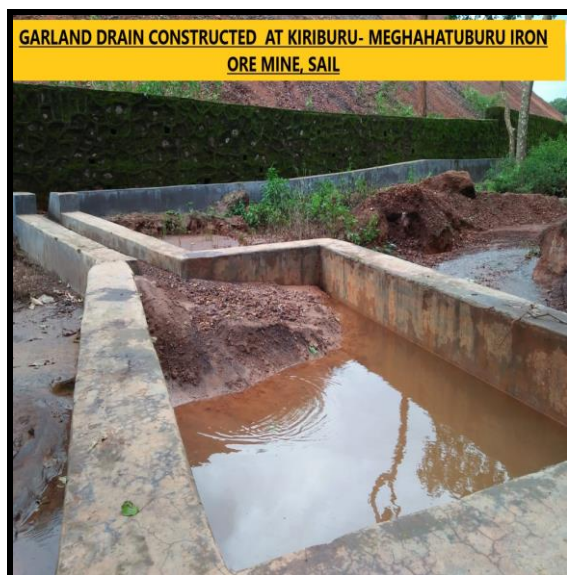
ANNEXURE-19: B- GARLAND DRAIN CONSTRUCTED AT MEGHAHATUBURU IRON ORE MINES, SAIL
