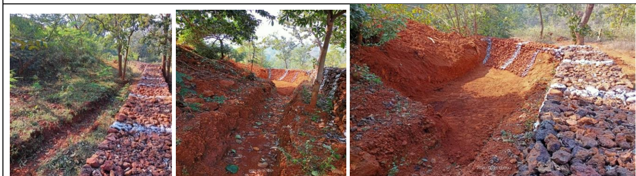
Garland Drain & Silting pond at Waste Dump-1
