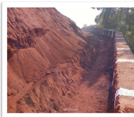
Desilting of Garland Drain at Fines Dump
