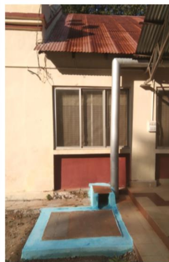
Roof top Rain Water Harvesting at Chiria Guest House
