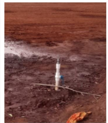
Laid of 360 m Water Supply with connector at Manoharpur Railway Siding Area
