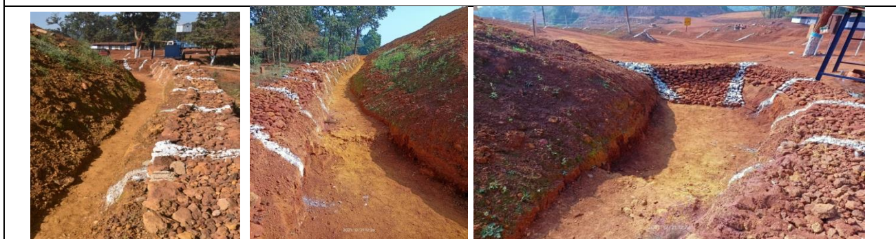
Garland Drain & Silting pond at Waste Dump-2
