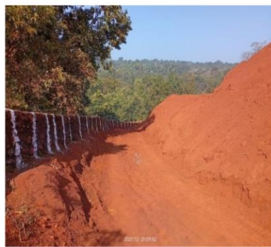
Desilting of Garland Drain at Fines Dump
