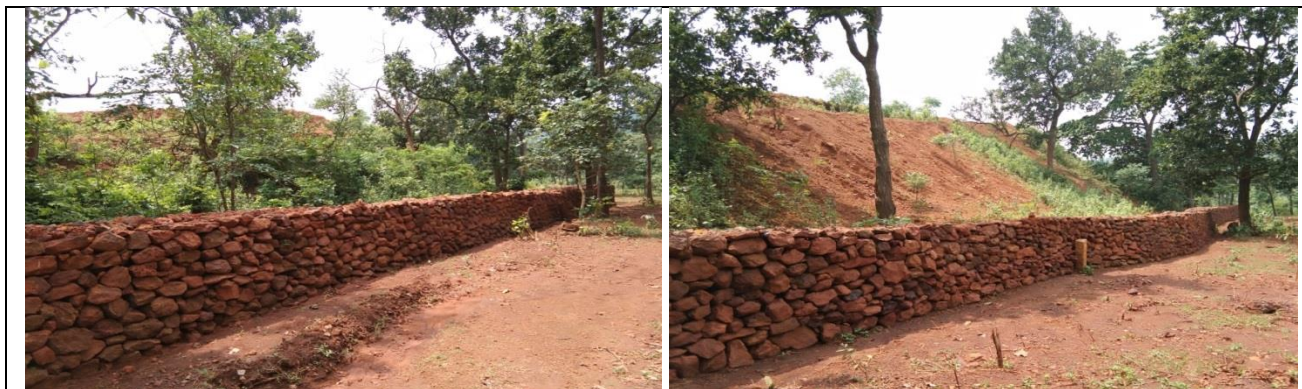
Retaining wall at Waste Dump-1
