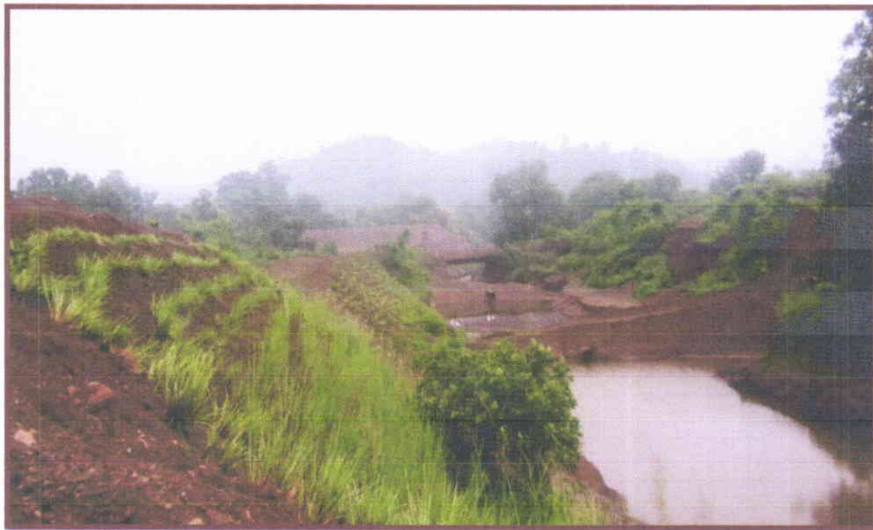
Photo: Settling cum Harvesting Pits along-with vetiver plantation near Zero Point Nalla
