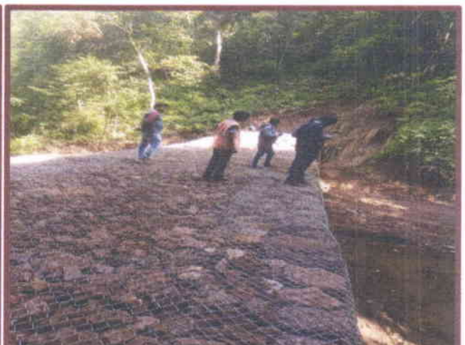
Photos: Construction of additional gabion boulder wall at the foot of Ranichua Waste Dump
