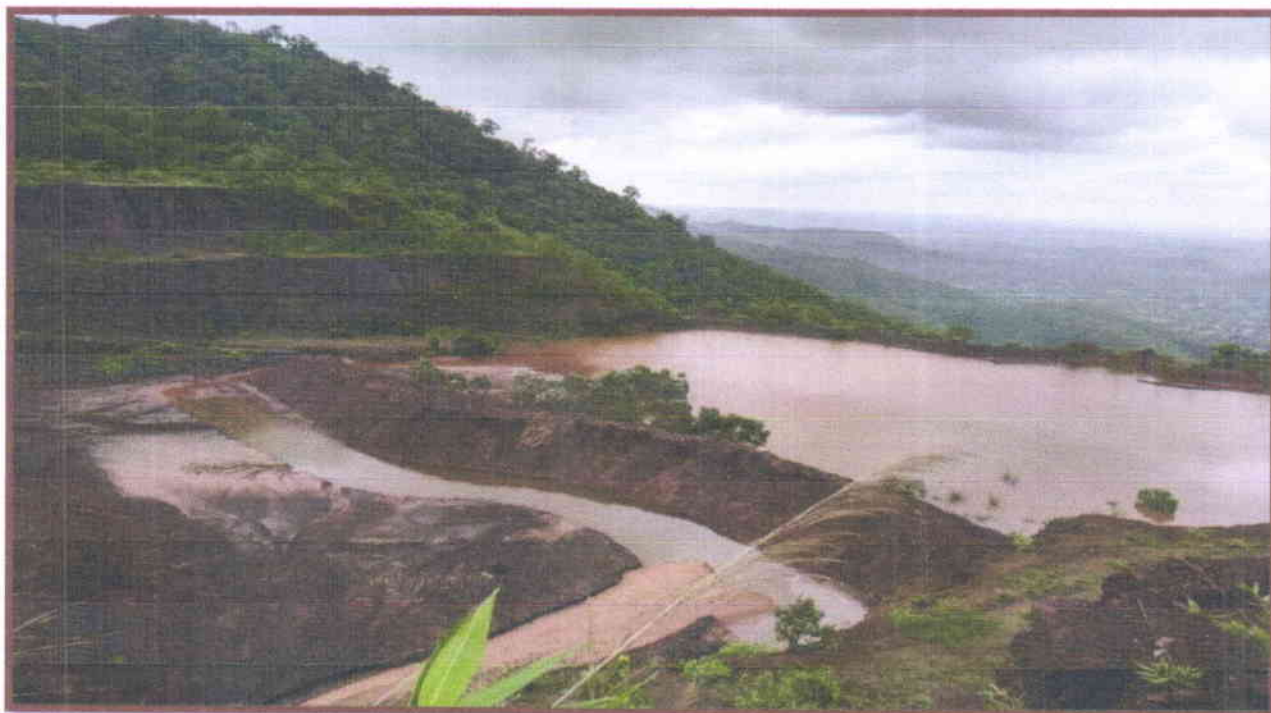
Photo: Rain Water Harvesting cum Settling Pond at IIInd Level Area of Mines
