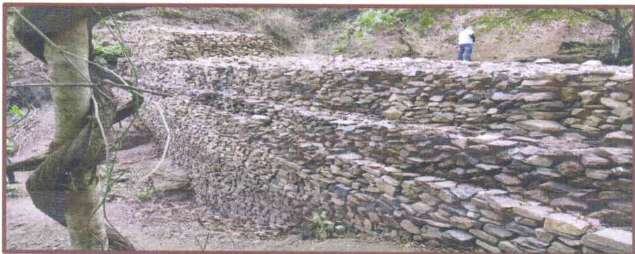
Photo: Boulder wall constructed at the toe of Ranichua waste dump area
