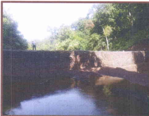
Photos: Construction of additional gabion boulder wall at the foot of Ranichua Waste Dump
