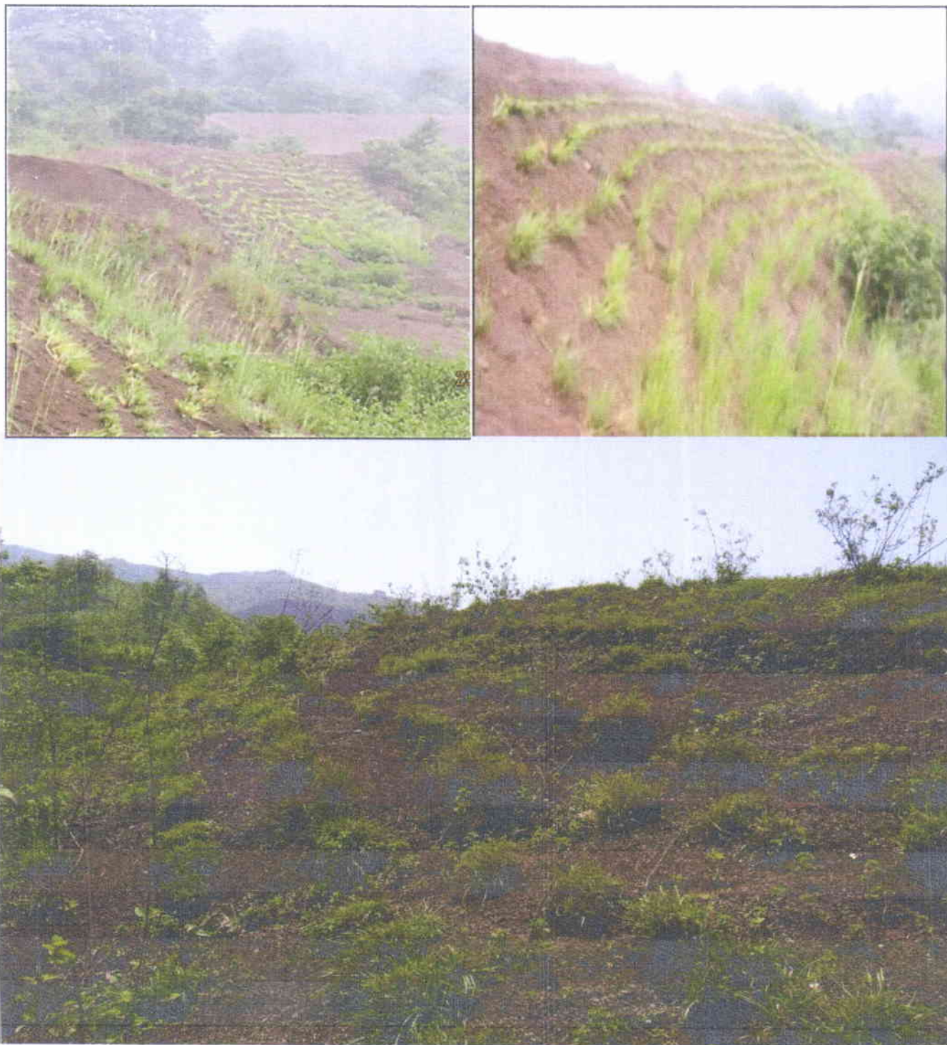
Photograph: Vetiver Plantation to bind the Soil at Slope of Sedimentation Traps
