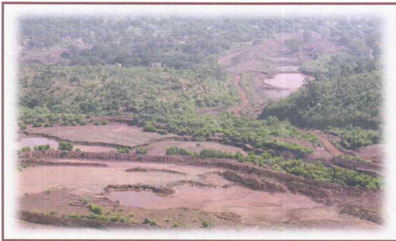
Photo: Earthen Dams and Sedimentation Traps at the slope of Fines Heap
