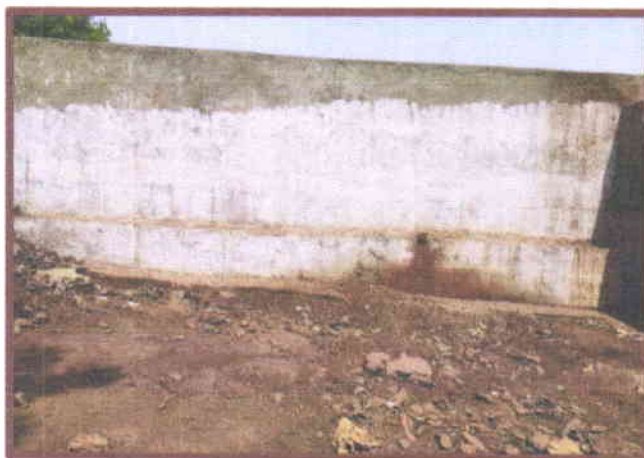
Photos: Construction of additional check dam at Zero point nalla & all opening in the dams are closed to restrict flow of water through it
