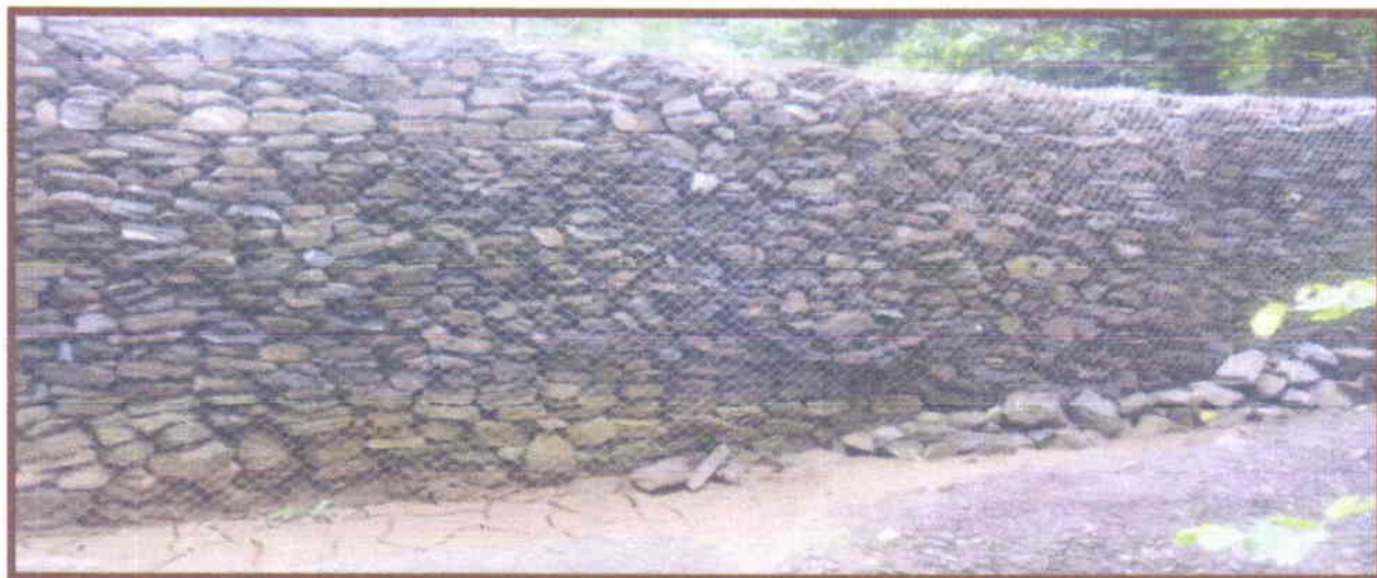
Photo: Boulder Wall the bottom of OT Hill Waste Dump
