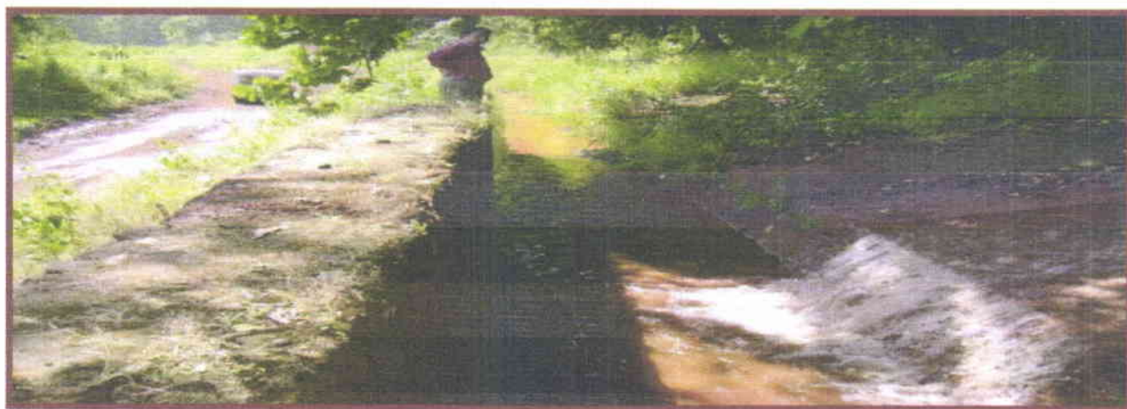
Photo: Garland Drain to divert runoff water into the pits
