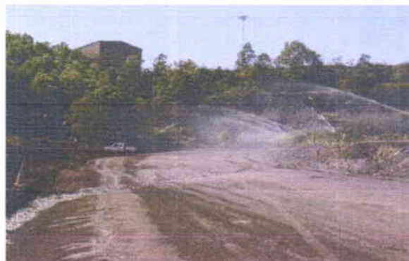
Photo: Permanent Road Sprinklers in Mines
