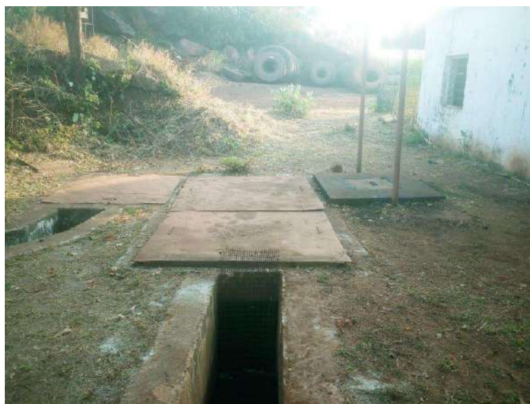
Oil & Grease trap at F/M Area, Barsua
