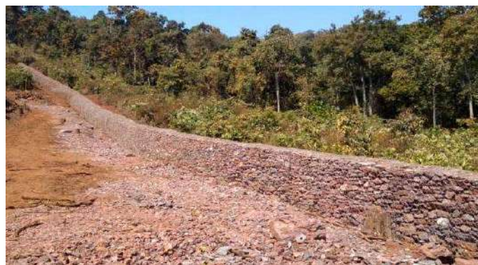
Dry Boulder wall at Waste Dump, Taldih
