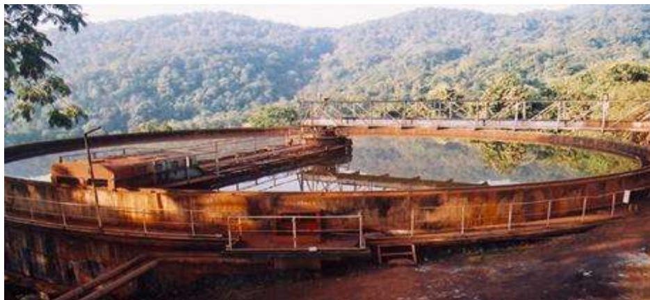
Thickener for Treatment of Effluent from Beneficiation Plant
