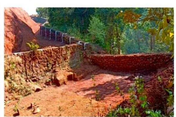
Check Dams across Nallahs to control Surface Runoff
