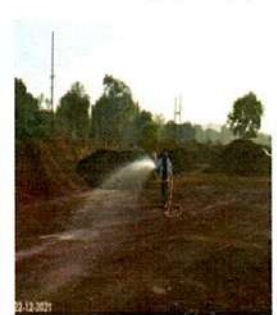
Water sprinkling system at Railway Siding Area by fixed water pipe line
