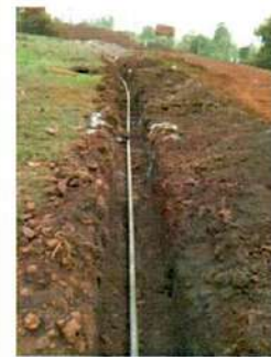
Water sprinkling system at Railway Siding Area by fixed water pipe line
