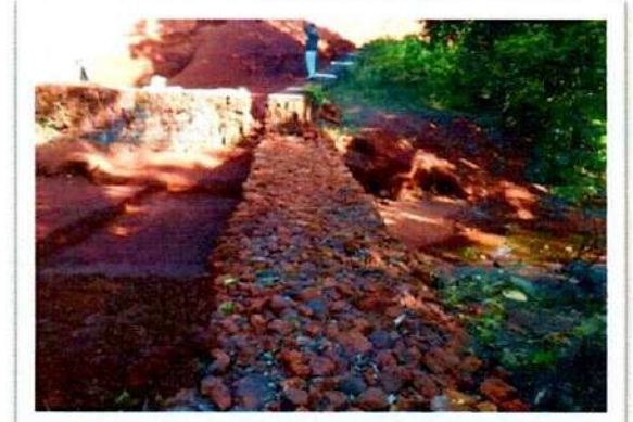
Check Dams across Nallahs to control Surface Runoff
