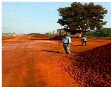
Water sprinkling at Railway Siding Area
