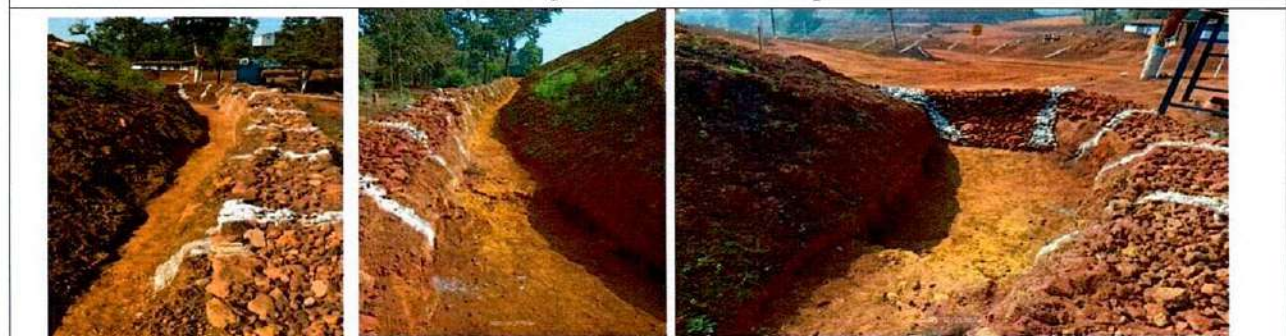
Garland Drain & Silting pond at Waste Dump-2
