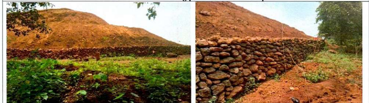
Retaining wall at Waste Dump-2
