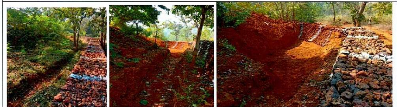
Garland Drain & Silting pond at Waste Dump-1
