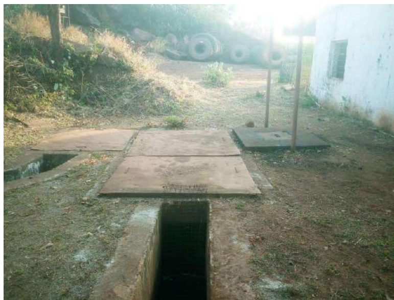
Oil & Grease trap at F/M Area, Barsua
