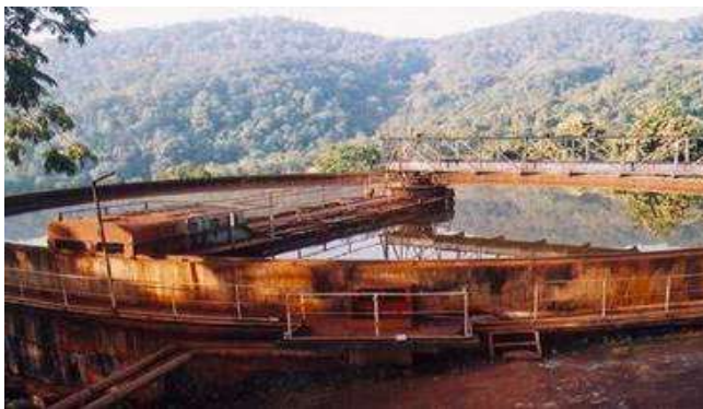
Thickener for Treatment of Effluent from Beneficiation Plant
