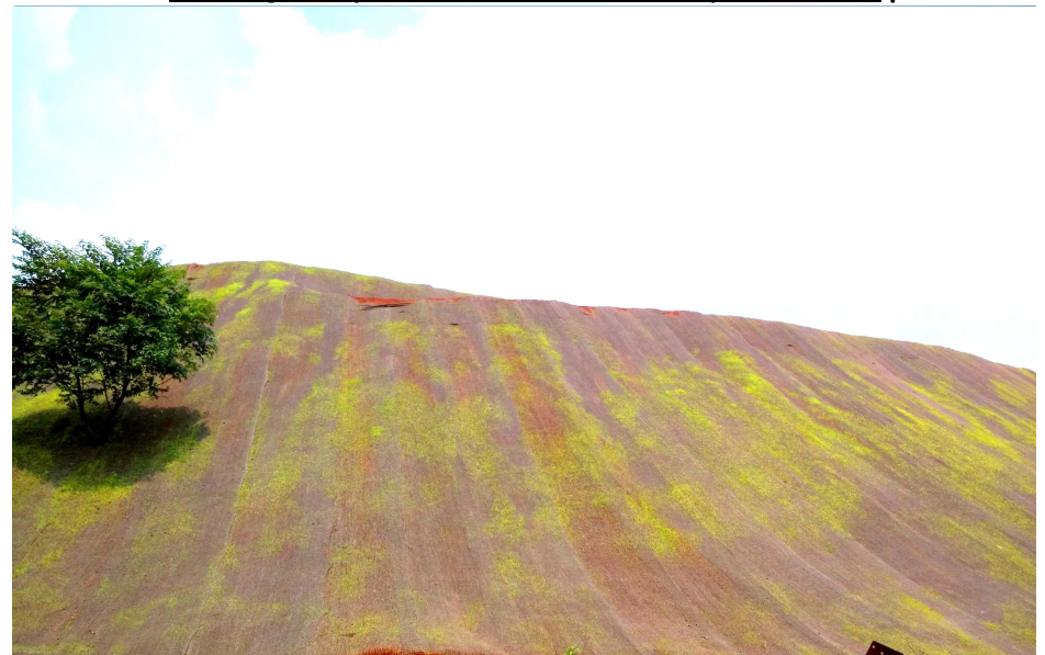
Coir Matting on DH-5 subgrade dump
