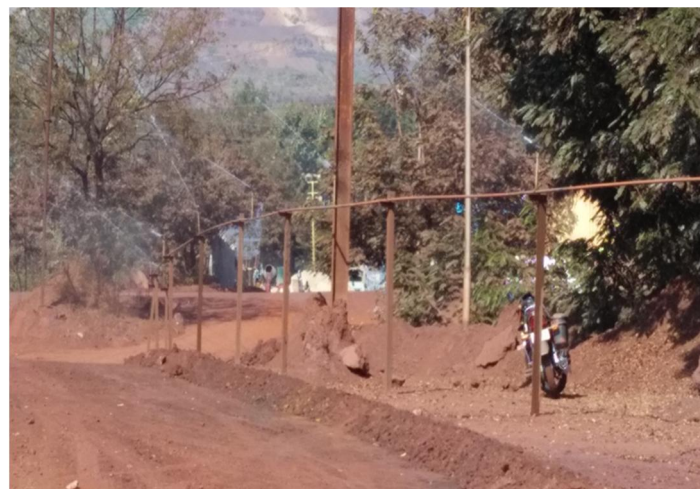
Photograph showing water sprinkling system on Haul Road near 600 TPH Plant
