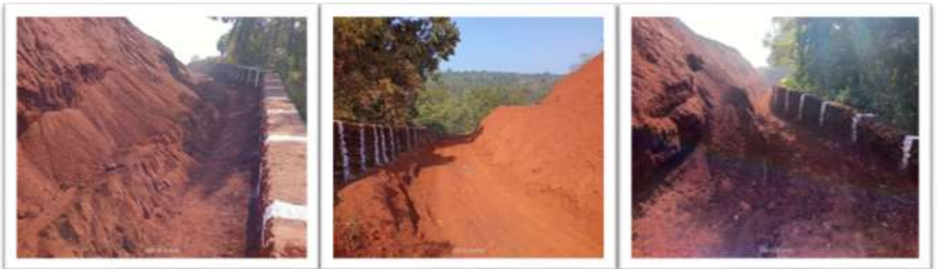
De-silting of Garland Drain at Fines Dump
