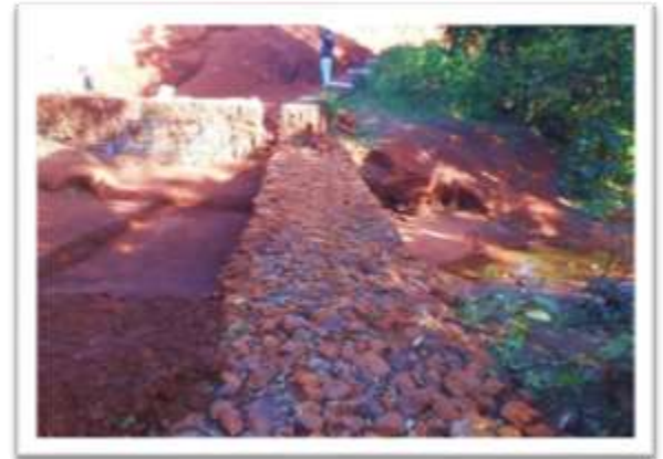
Check Dams across Nallahs to control Surface Runoff
