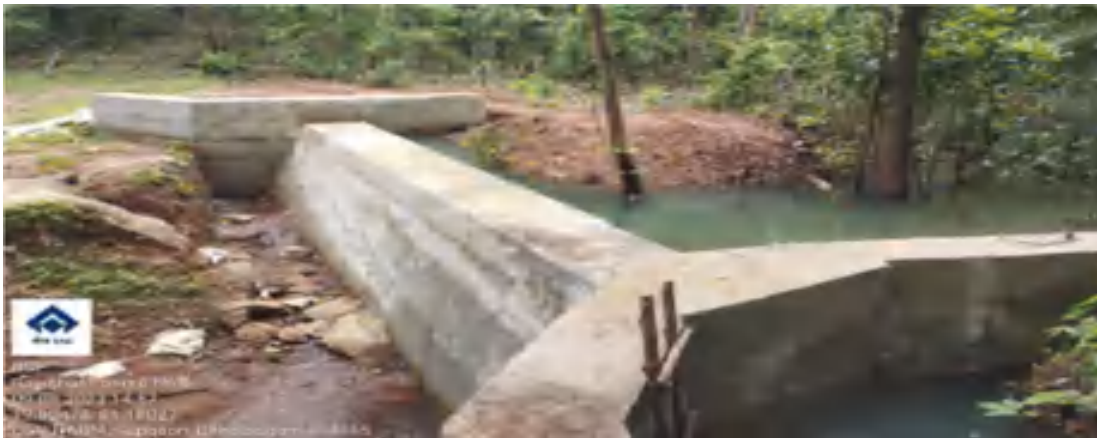
Concrete Dam at the foot hill
