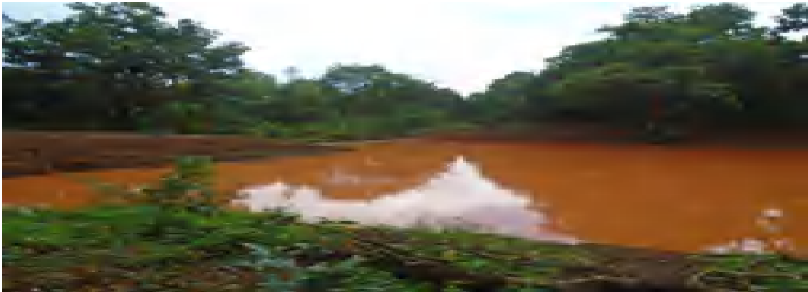
View of Check dam, constructed as part of rain water harvesting measures.
