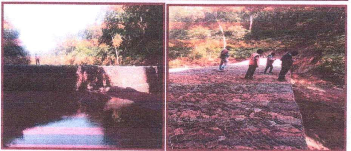
Photo: Construction of additional gabion boulder wall at the foot of Ranichua Waste Dump
