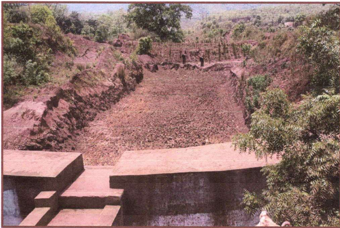
Photo: Desiltation near Zero Point check dam and earthen traps.
