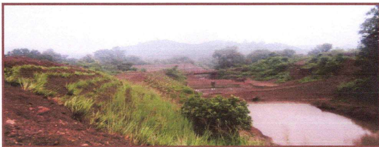
Photo: Settling cum Harvesting Pits along-with vetiver plantation near Zero Point Nalla
