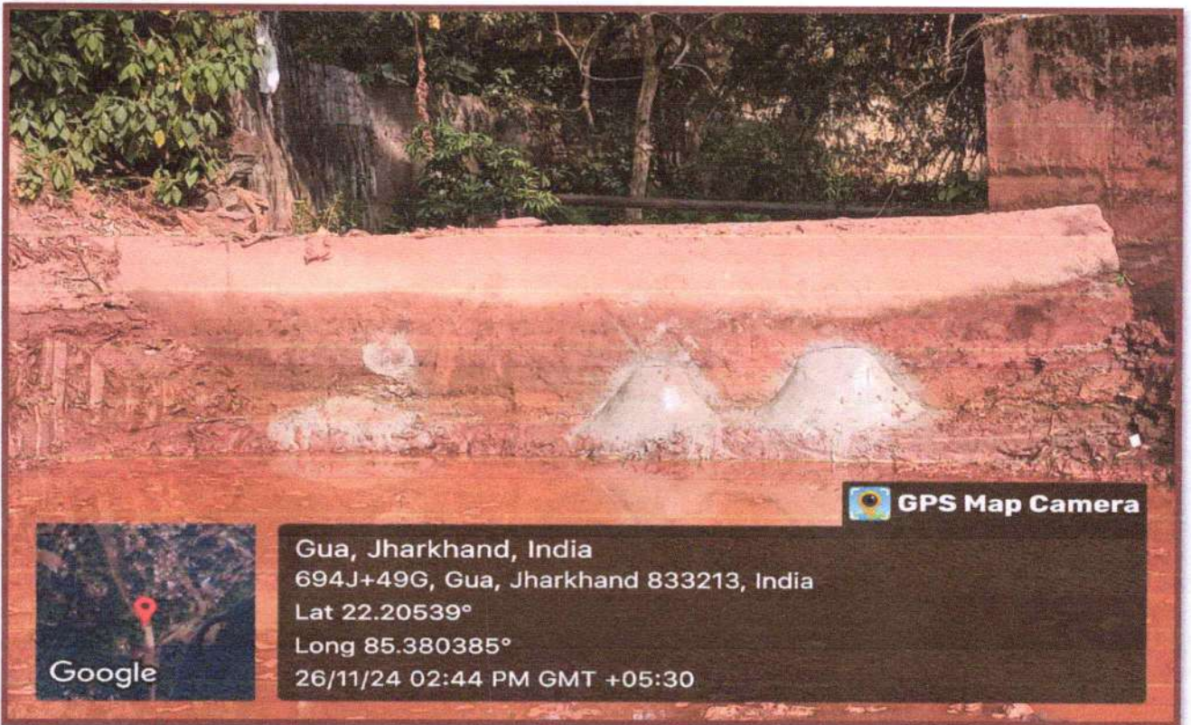
Photo: Desiltation of Kalimandir Check Dam and closing of hole completed.
