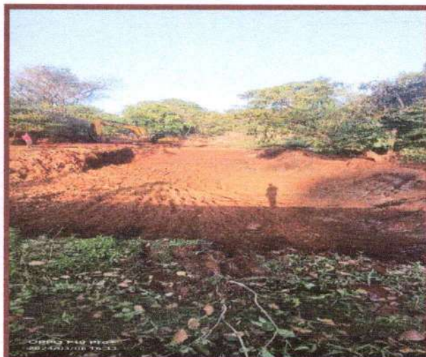
Photos: Desiltation at u/s side of Check Dam near Kali Mandir & Gojapahar Nalla
