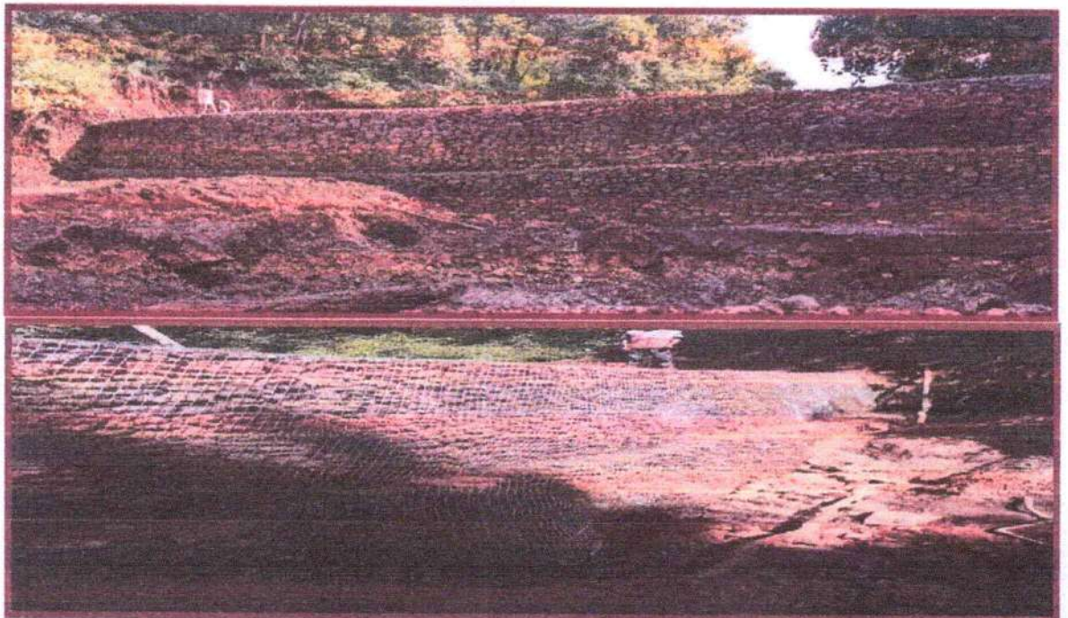
Photo: Settling cum Harvesting Pits along-with vetiver plantation near Zero Point Nalla
