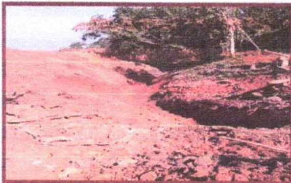
Photo: Garland Drain to divert runoff water into the pits
