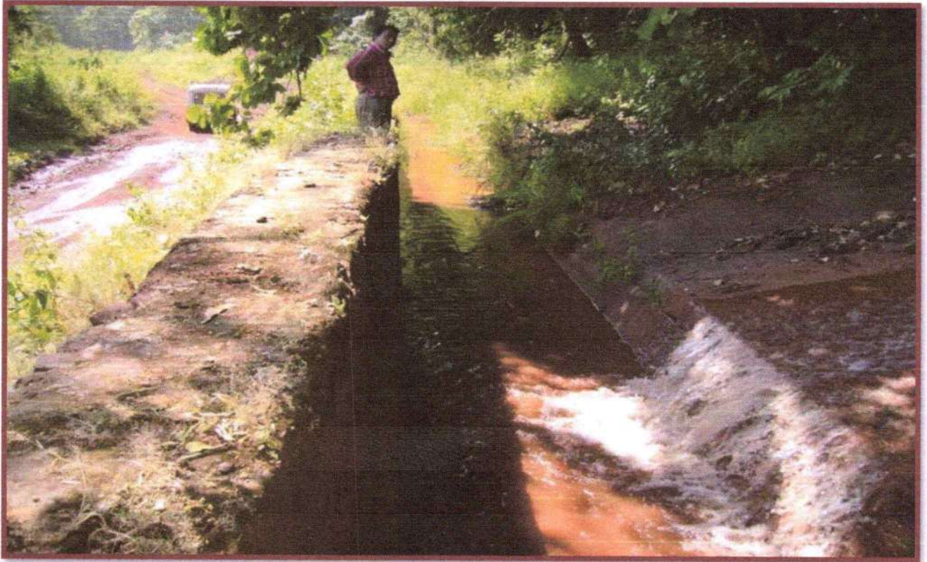
Photo: Garland Drain to divert runoff water into the pits
