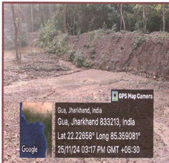
Photos: Newly constructed Sedimentation cum rainwater harvesting pond at foot of OT Hill Waste dump area.
