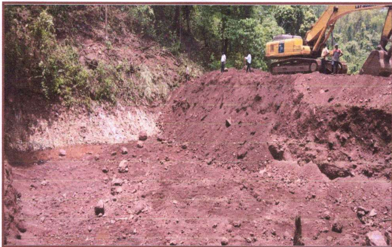
Photos: Newly constructed Sedimentation cum rainwater harvesting pond at foot of Ranichua waste dump area.
