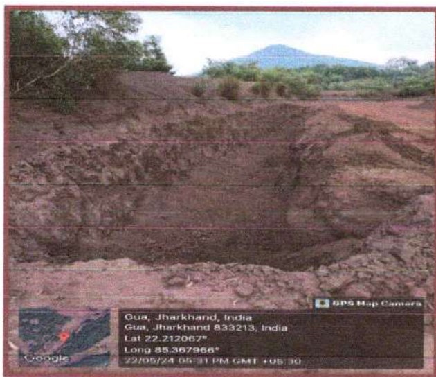
Photos: Settling Pits / Sediment Traps constructed between Dam 1, 2 and 3 to control flow of fines
