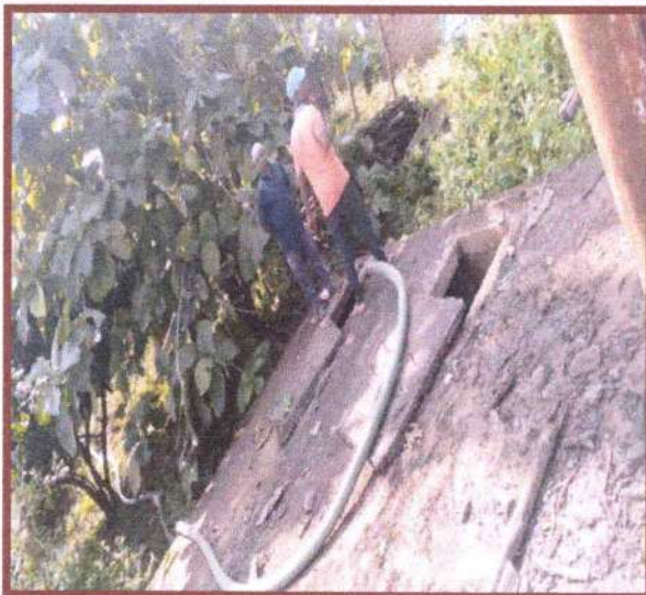
Photographs showing Septic tanks and its cleaning through mechanical mode
