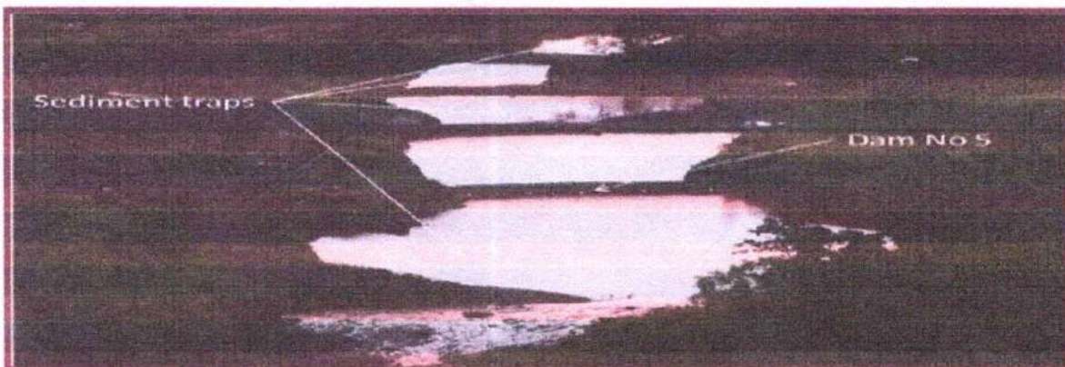
Photo: Series of 5 nos. of earthen dams followed by 4 nos. of settling ponds at the foot of Fines Heap
