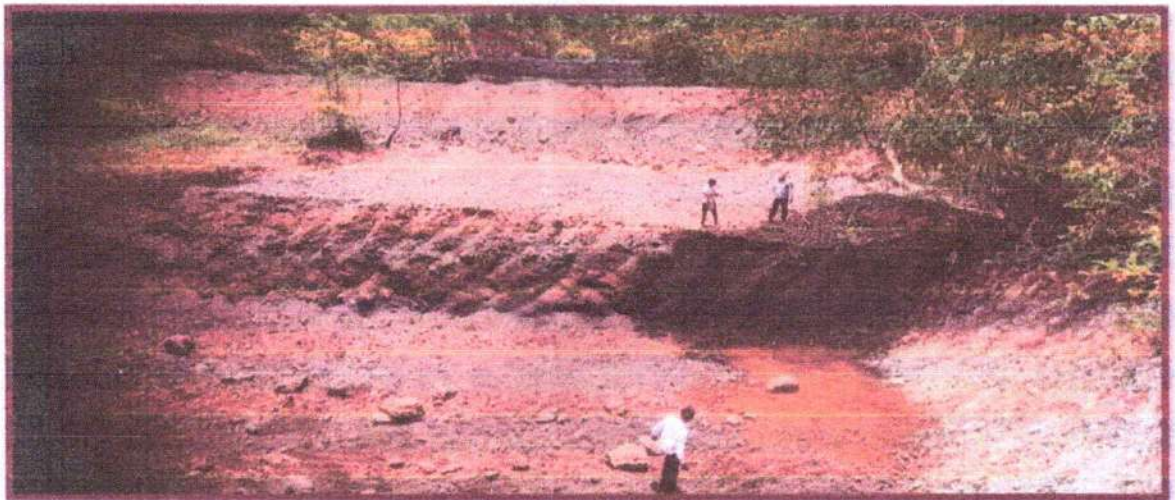
Photos: Newly constructed Sedimentation cum rainwater harvesting pond at foot of Ranichua waste dump area.
