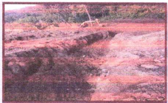
Photo: Boulder wall constructed at the toe of Ranichua waste dump area
