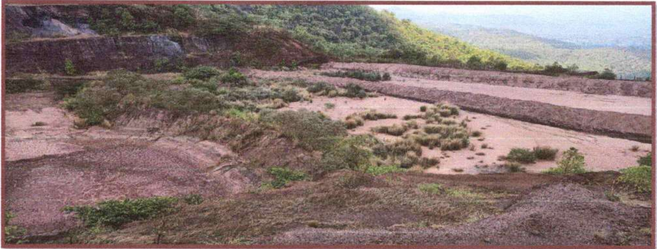
Photos: Rain Water Harvesting cum Settling Pond at IInd Level Area of Mines and desiltation of the same carried out
