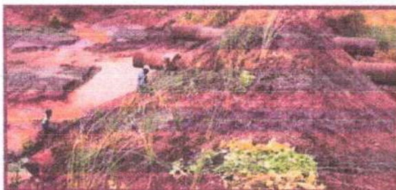
Photos: Plantation of local grass and hedge at slopes of earthen dam
