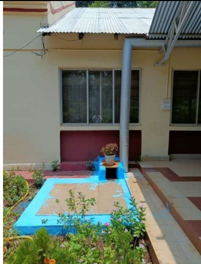
Roof top Rain Water Harvesting at Chiria Guest House
