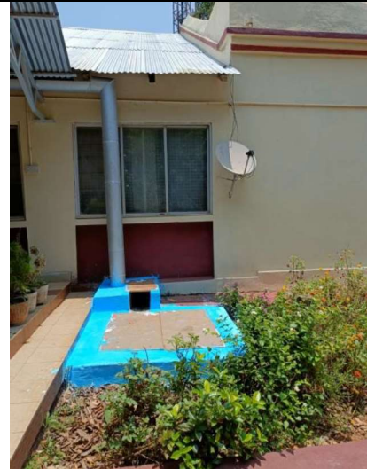
Roof top Rain Water Harvesting at Chiria Guest House
