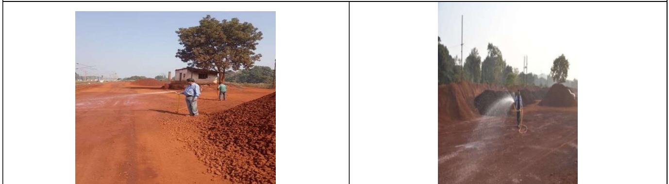
Water sprinkling at Railway Siding Area
