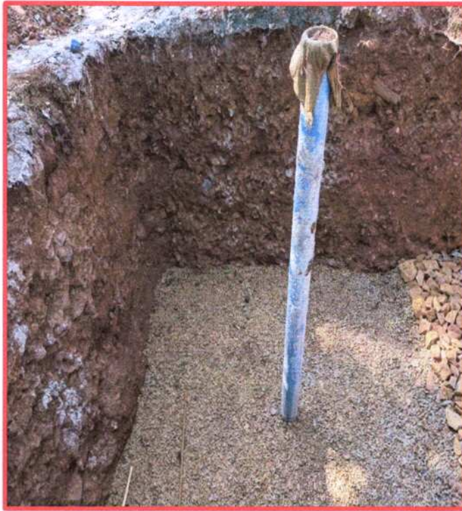
Photos: Photos of recharge pit cum shaft during construction period
