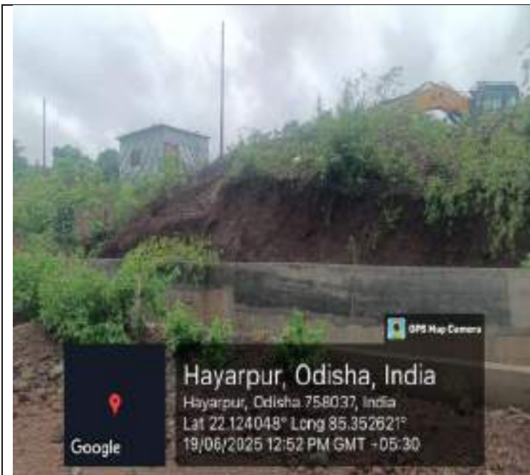
Retaining Wall and Garland Drain at Quarry-5
