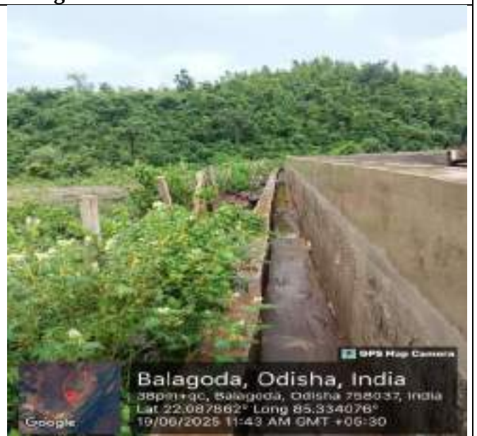
Retaining Wall and Garland Drain at Quarry-10
