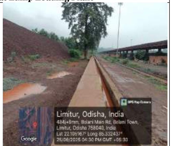
Retaining wall and Garland Drain at Lump Loading Plant
