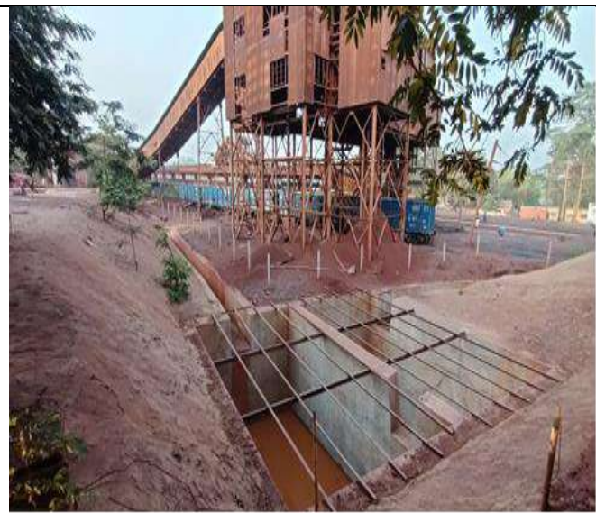
Settling Pits along with diverting drains to Handle surface Runoff from Lump Loading Plant
