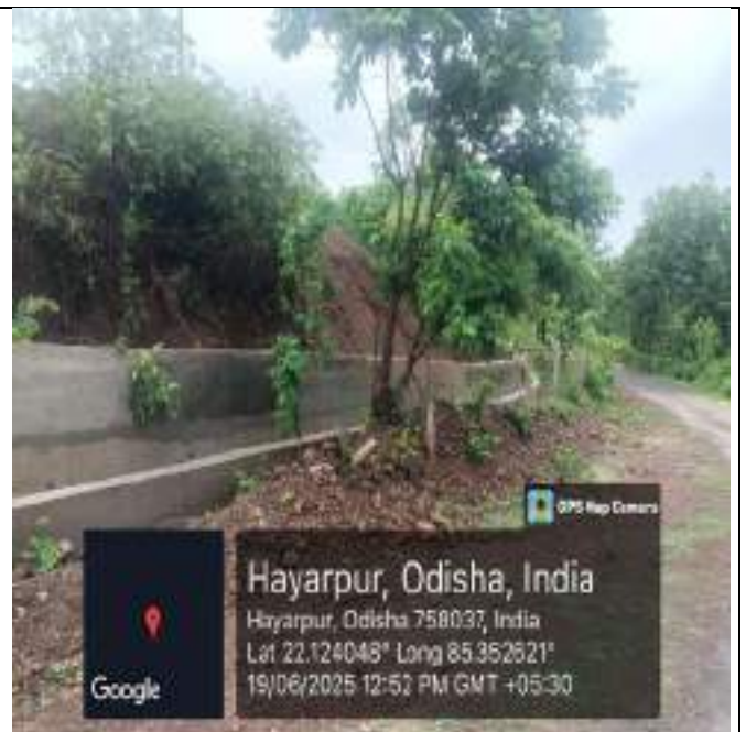
Retaining Wall and Garland Drain at Quarry-5
