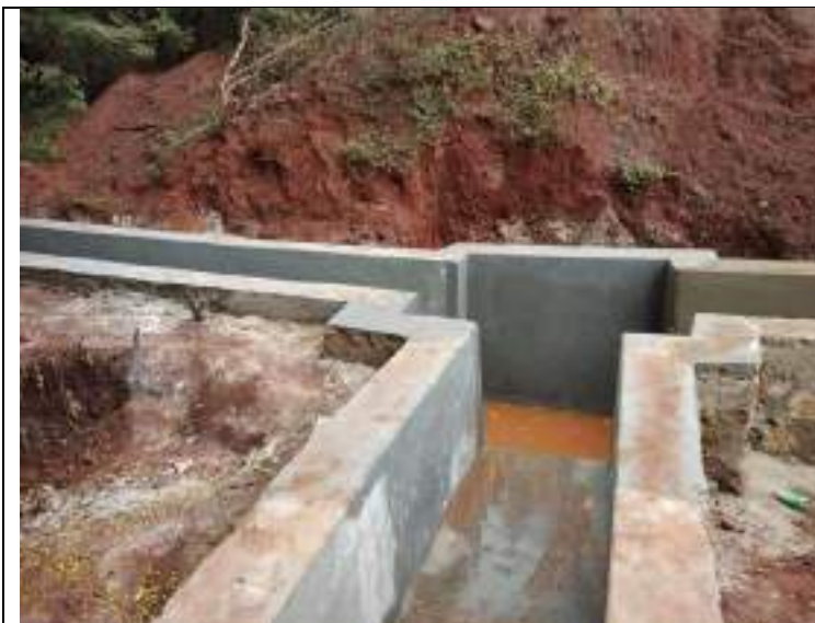
Settling Pits along with diverting drains to Handle surface Runoff from Lump Loading Plant
