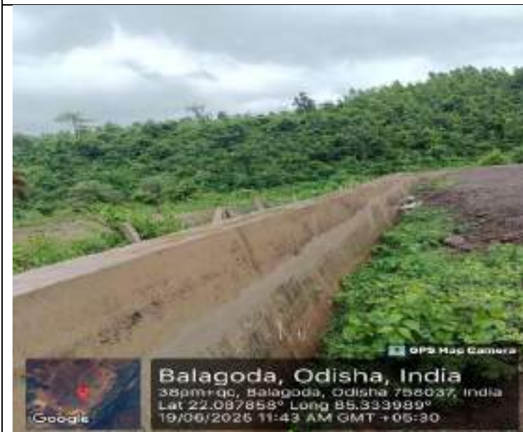
Retaining Wall and Garland Drain at Quarry-10
